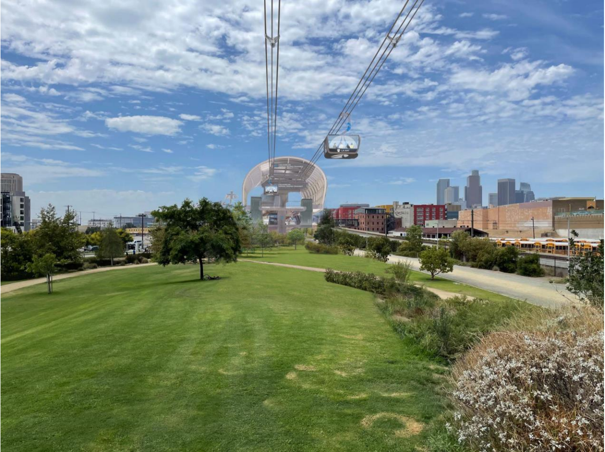
Figure 5-19b: Simulation View of KOP 16b – Looking Southeast from the Southwestern Portion of Los Angeles State Historic Park (View provided with 2 inch diameter haul rope (center rope) and 2.5 inch diameter track ropes)
