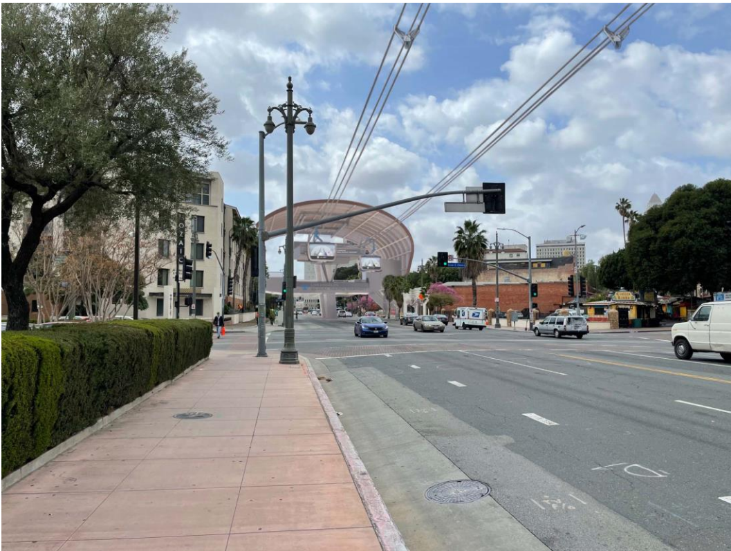
Figure 5-9: Existing and Simulation Views of KOP 8 – Looking South on Alameda Street from just North of Cesar Chavez Avenue
