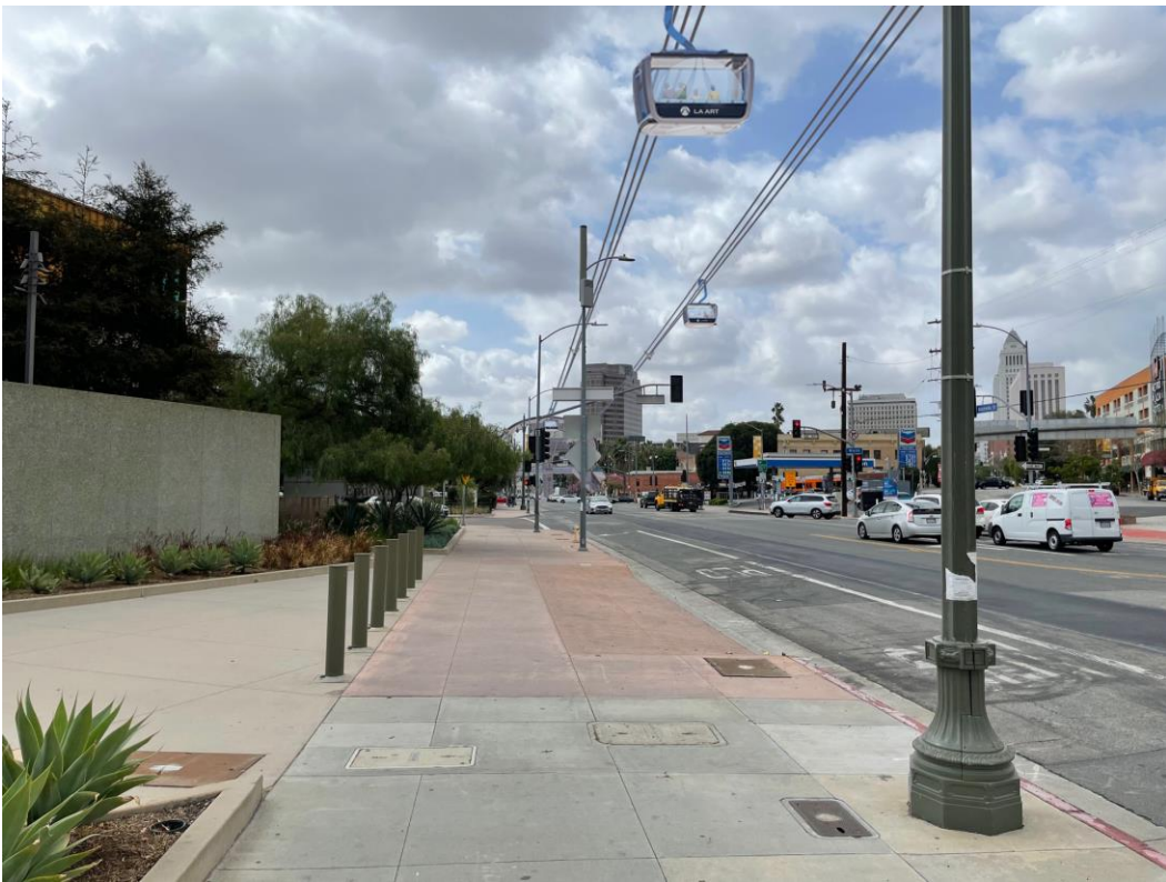
Figure 5-11: Existing and Simulation Views of KOP 10 – Looking South on Alameda Street at Main Street
