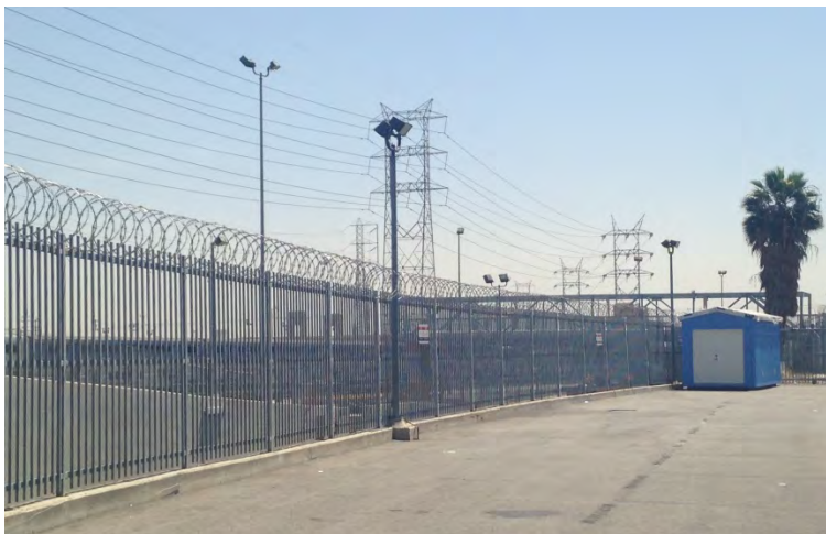
Facing south along north edge of project site
