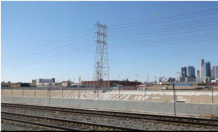
Facing south west from across LA River
