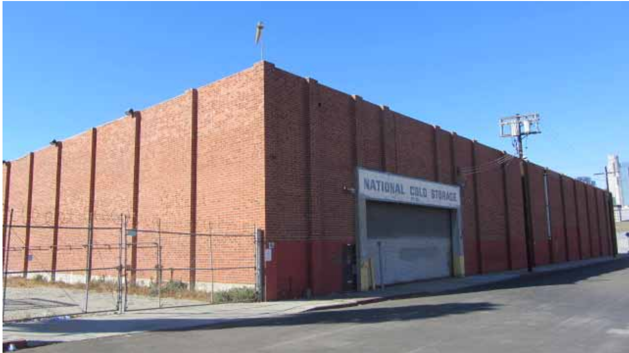
Plate 6: 820 E. Jackson Street, from Jackson Street, View Southwest
