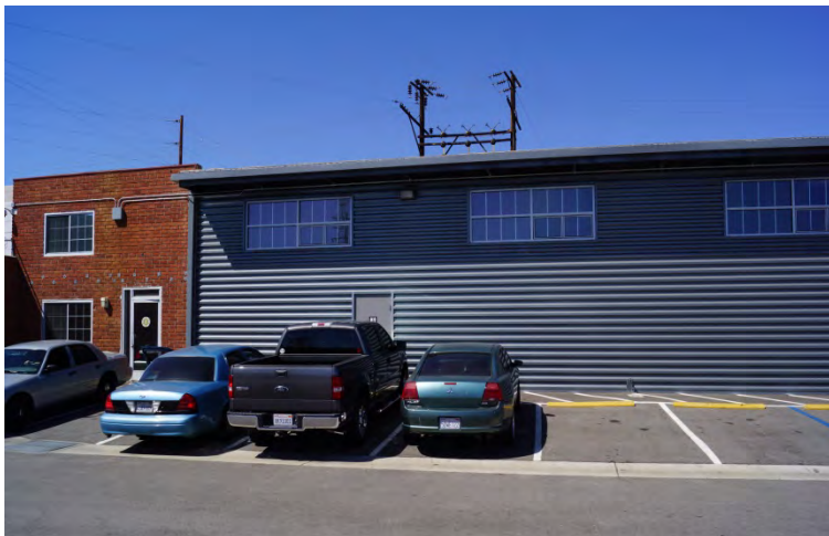
Existing Sherriff's building
