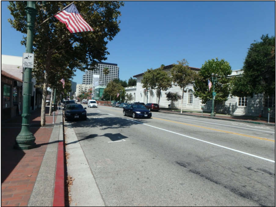
Photograph 17 – Intersection of East Broadway and South Kenwood Street along Curb-Running Configuration. View to the West.
