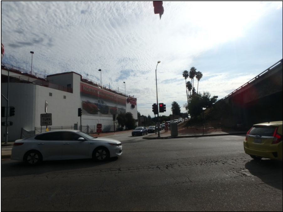
Photograph 8 – Intersection of Lankershim Boulevard and State Route 134 along Freeway-Running Configuration. View to the Northeast.
