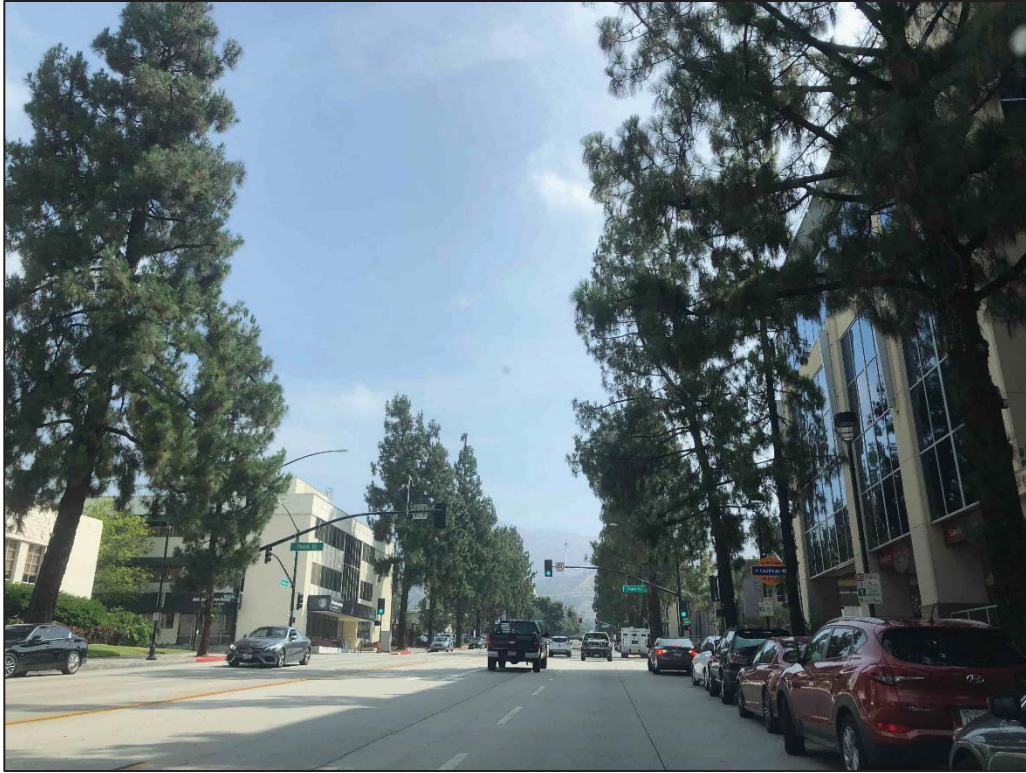
Photo 7. Proposed Bus Route, Olive Avenue and Third Street, View Facing East
