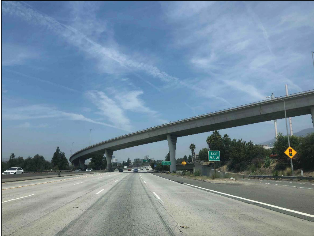
Photo 25. Proposed Bus Route, Westbound SR-134, View Facing West
