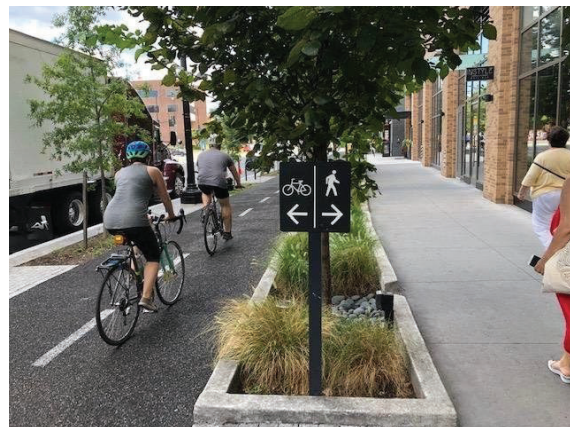
Example of raised bikeway showing physical barrier
