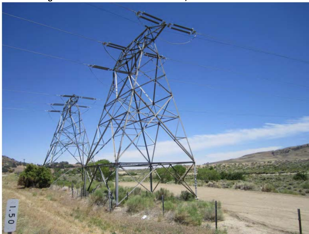
Big Creek East-West Transmission Line, view towards the east
