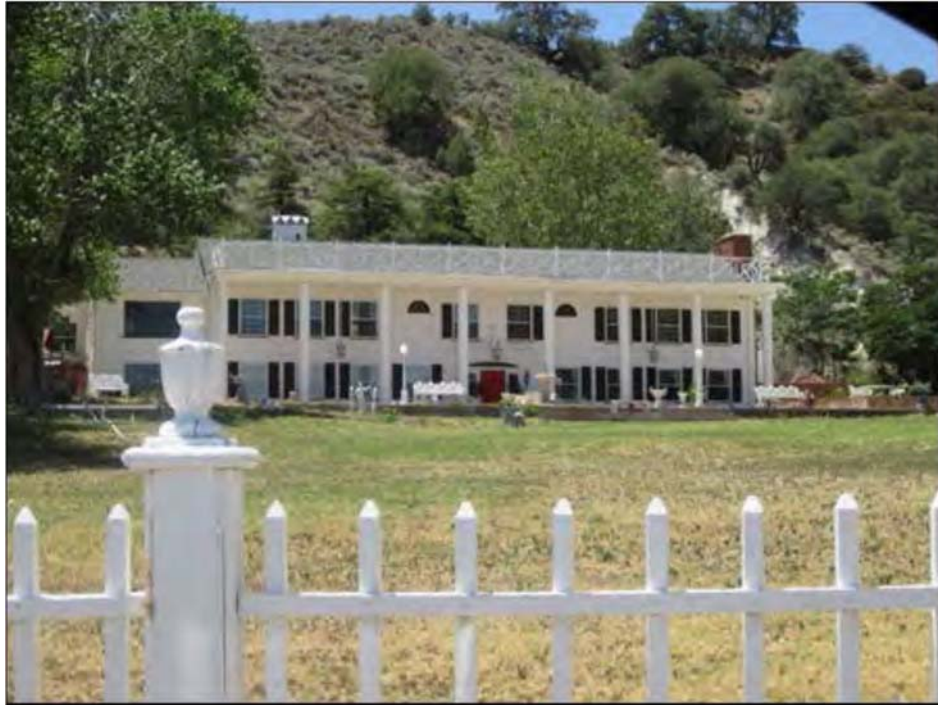
Kinsey Mansion façade and lawn, view from SR-138 towards the south
