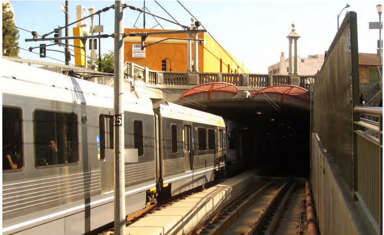
Metro Gold Line – Pasadena Tunnel near Colorado Boulevard
