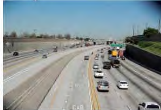
Metro Express Lanes Project I-10 and I-110 Freeways
