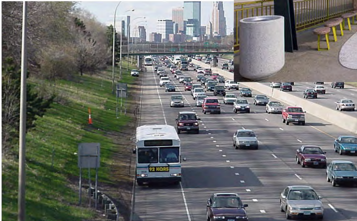
Freeway with Shoulder Running BRT - Minneapolis
