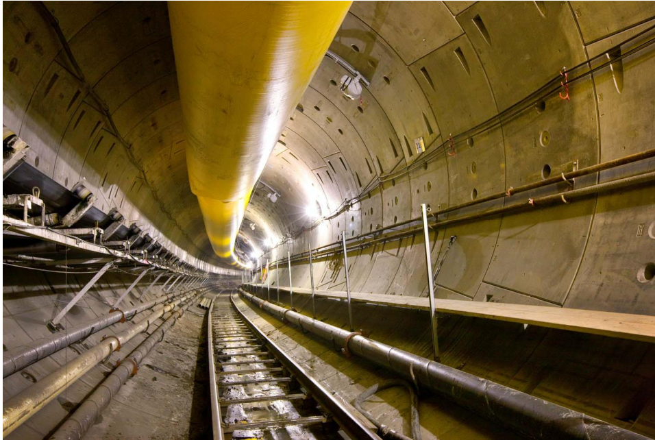
Figure 6-5. Precast Concrete Segmental Lining, University-Link LRT Tunnel
