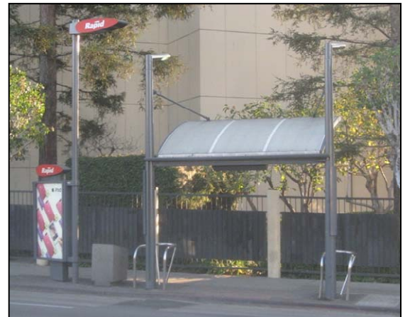
FIGURE 11 Metro Rapid Station and Shelter
