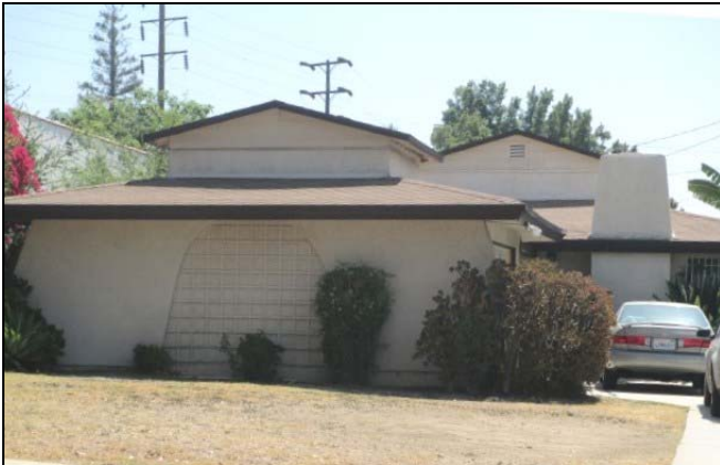
4536 Maycrest Avenue (APE Map Ref # 158-3A). View to the east.
