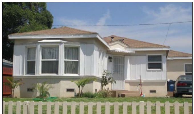
3211 Front Street. View to the north.
