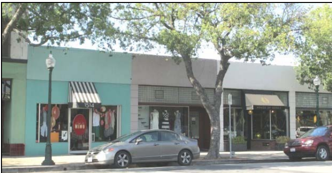
1514-1522 Mission Street (west bays). View to the north.
