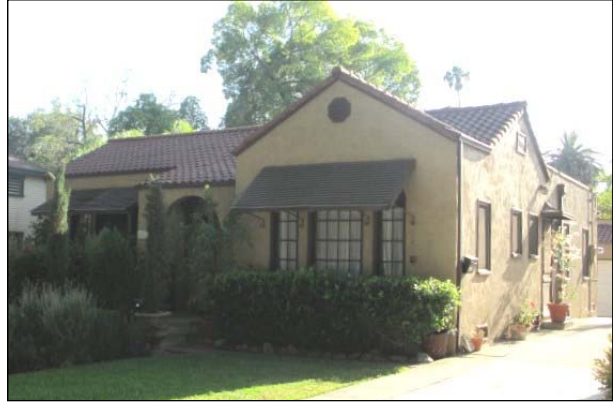
1017 Diamond Avenue (APE Map Ref # 304-3A). View to the southwest.
