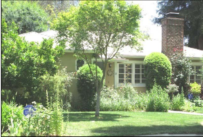
308 Fairview Avenue (APE Map Ref # 384-3A). View to the southeast.
