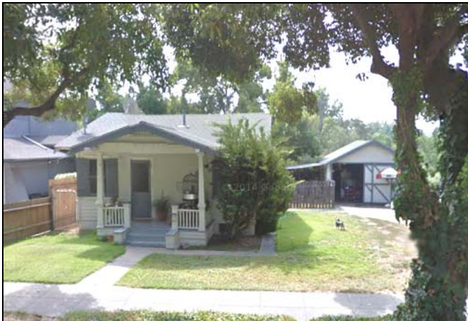
1035 Foothill Street (APE Map Ref # 263-CT-3A). View to the south (Google 09/2011).
