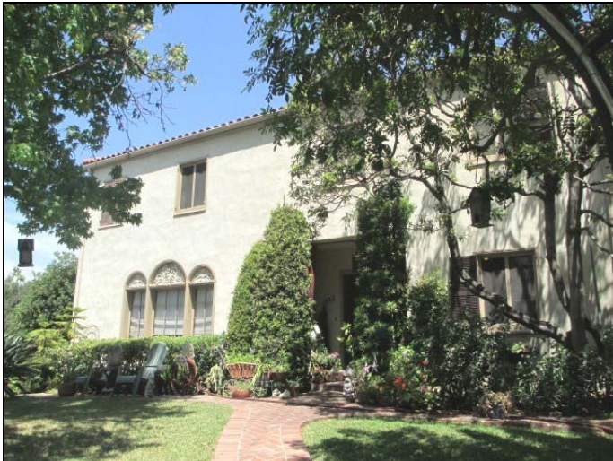
1332 El Cerrito Circle. View to the northeast.
