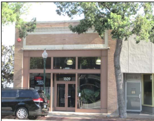
1509 Mission Street. View to the south.
