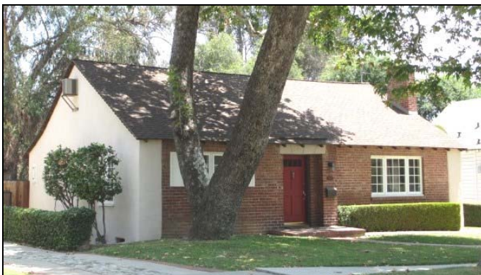
300 Fairview Avenue (APE Map Ref # 387-3A). View to the southeast.
