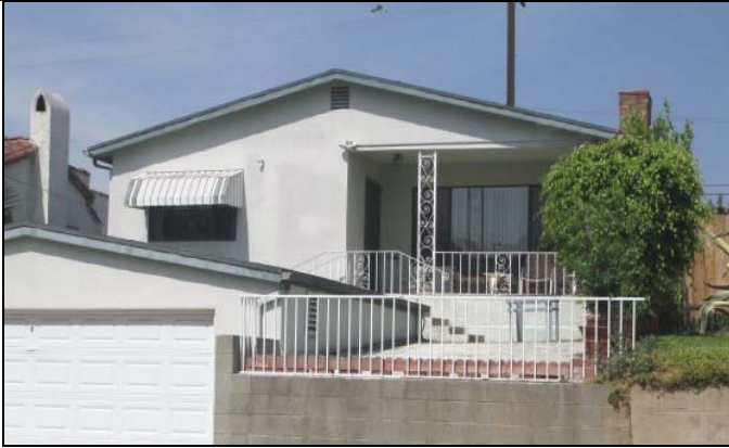
1643 Westmont Drive. View to the west.
