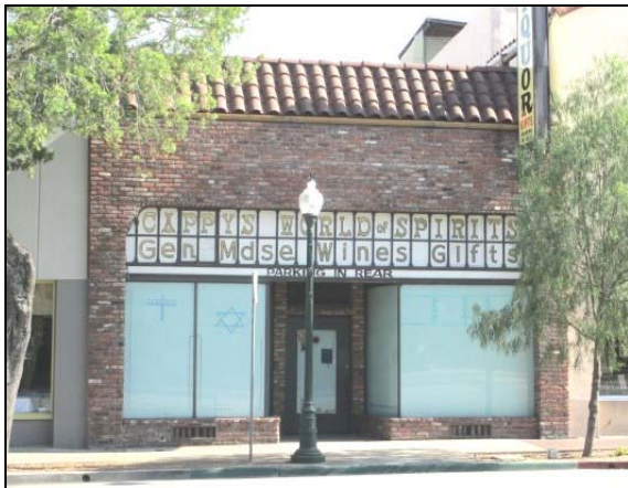
1503 Mission Street. View to the south.
