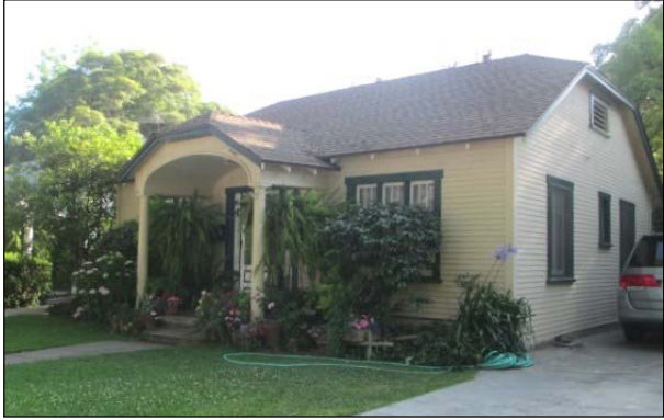
1021 Diamond Avenue (APE Map Ref # 302-3A). View to the southwest.
