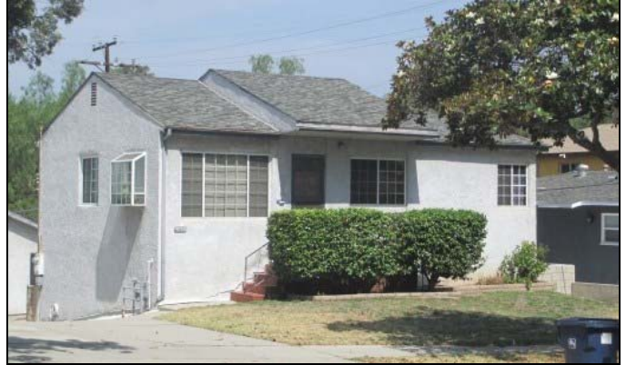
1717 Westmont Drive. View to the west.
