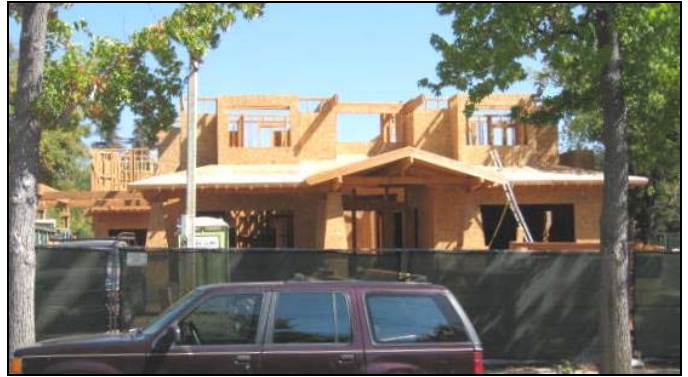
402 Fairview Avenue. View to the east (taken 10/02/13).
