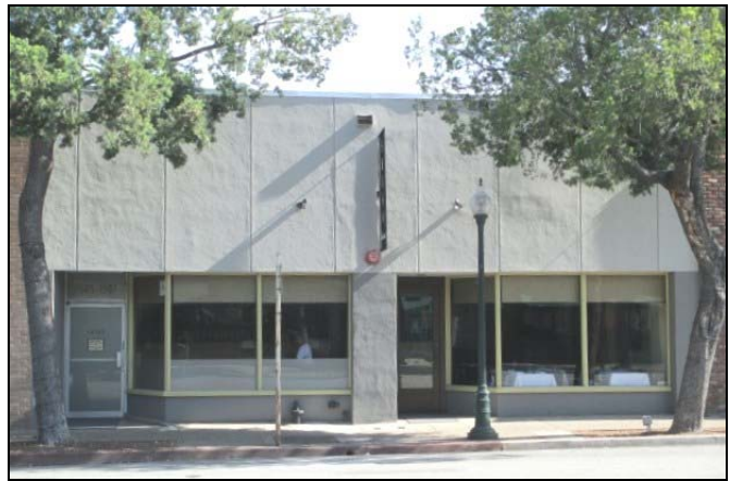
1505-07 Mission Street. View to the south.
