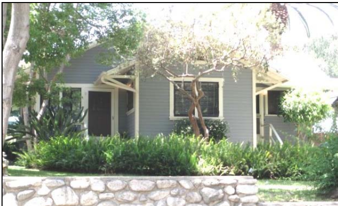
225 Fairview Avenue (APE Map Ref # 270-CT-3A). View to the west.
