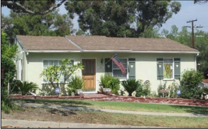
1721 Westmont Drive. View to the west.
