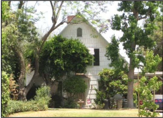
330 Fairview Avenue (APE Map Ref # 378-3A). View to the east.
