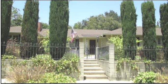
1030 Highland Street. View to the north.
