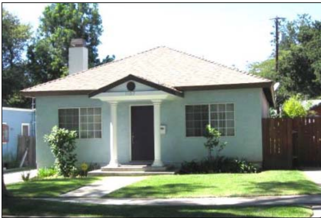
1107 Diamond Avenue. View to the west (taken 10/1/13)
