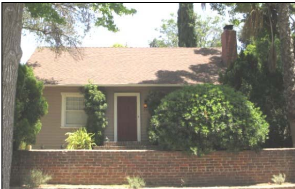
316 Fairview Avenue (APE Map Ref # 382-3A). View to the east.
