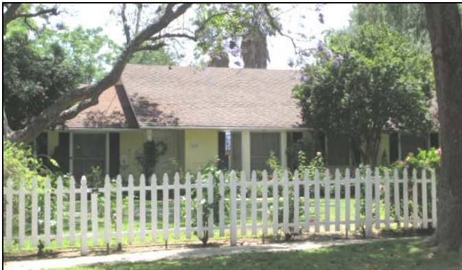
1033 Buena Vista Street (APE Map Ref # 369-3A). View to the south.
