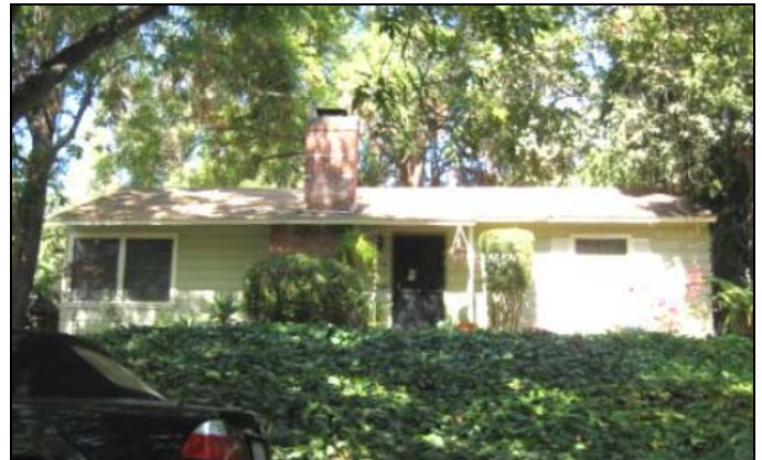
1038 Foothill Street (APE Map Ref # 364-3A). View to the north (taken 10/2/13).
