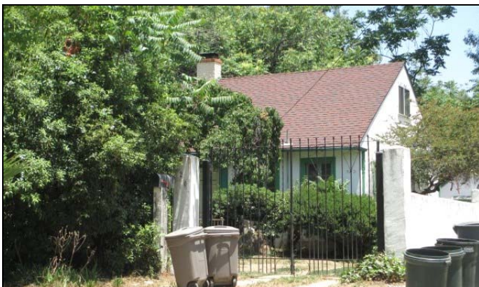
320 Fairview Avenue (APE Map Ref # 380-3A). View to the northeast.
