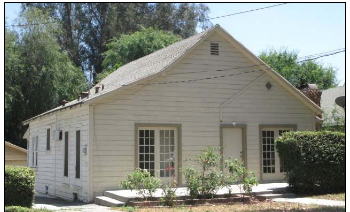
302 Fairview Avenue (APE Map Ref # 272-CT-3A). View to the southeast.
