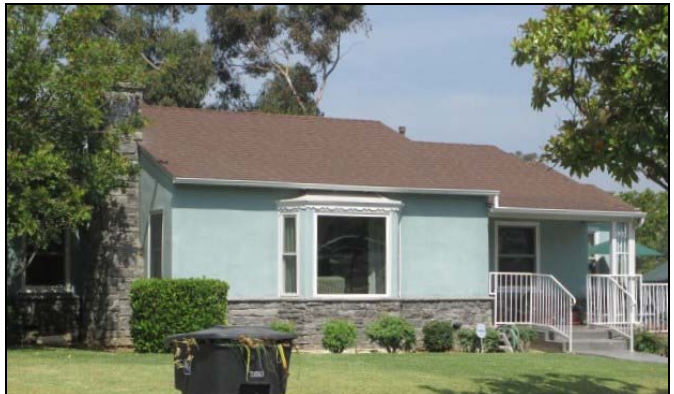
1805 Westmont Drive. View to the west.
