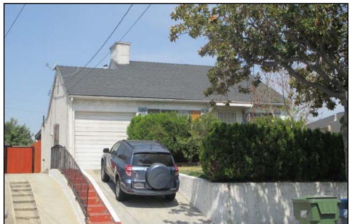
1619 Westmont Drive. View to the west.
