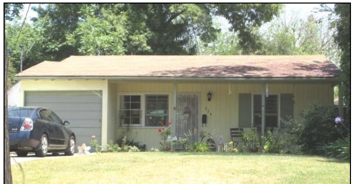
328 Fairview Avenue (APE Map Ref # 379-3A). View to the east.
