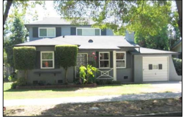
1039 Foothill Street. View to the south (taken 10/2/13)
