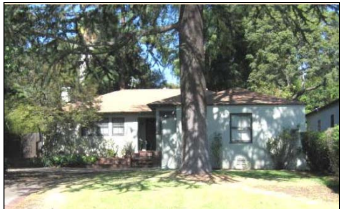
1020 Foothill Street (APE Map Ref # 361-3A). View to the north (taken 10/2/13).
