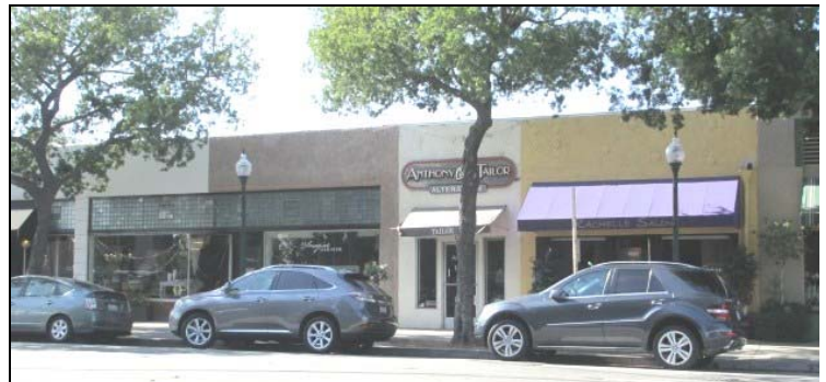
1514-1522 Mission Street (east bays). View to the north.
