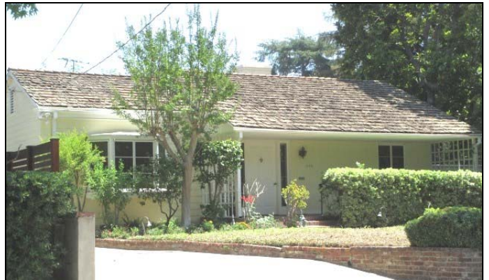
414 Fairview Avenue (APE Map Ref # 375-3A). View to the southeast.
