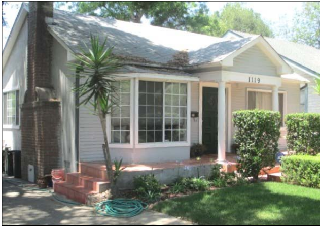
1119 Diamond Avenue. View to the northwest.
