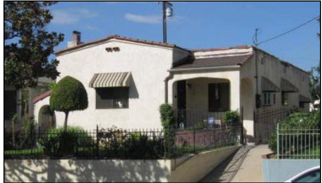
1625 Westmont Drive. View to the southwest (taken 9/26/13).
