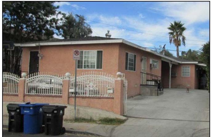
4343 Winchester Avenue. View to the west (taken 10/07/13).
