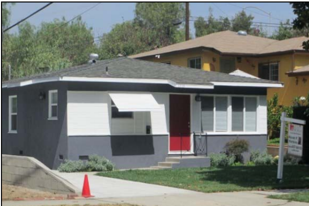
1715 Westmont Drive. View to the west.
