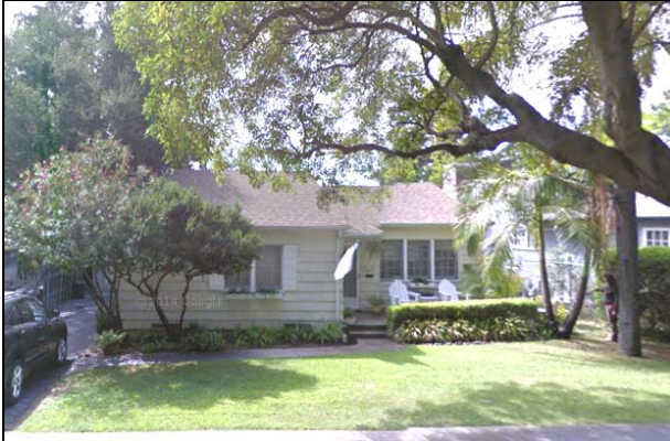
1041 Foothill Street (APE Map Ref # 264-CT-3A). View to the south (Google 09/2011).
