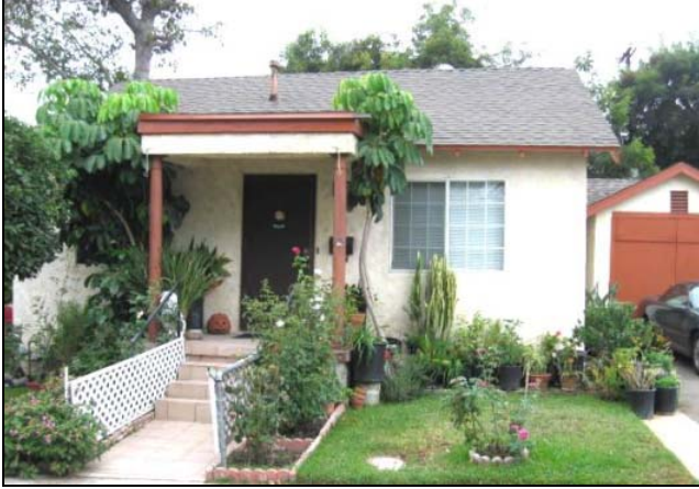
725 Hope Court. View to the west (taken 10/2/13).
