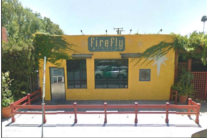
1009 El Centro Street (altered property; view to the south; Google 2015)
