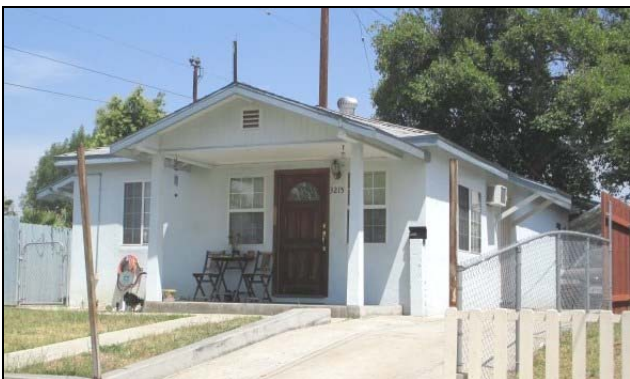
3215 Front Street. View to the north.
