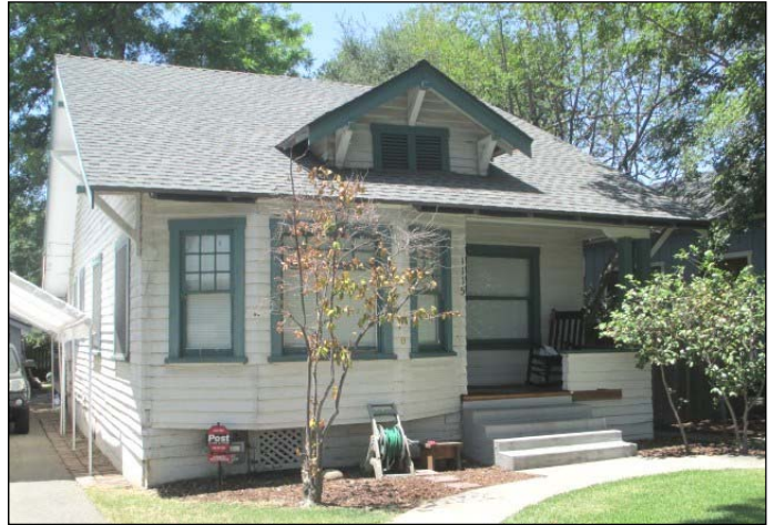
1115 Diamond Avenue (APE Map Ref # 289-3A). View to the northwest.
