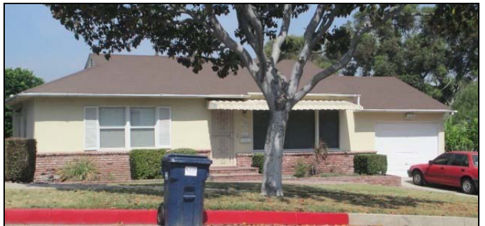
1725 Westmont Drive. View to the west.
