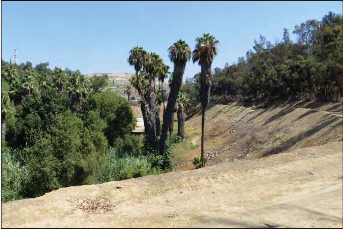
Photo A of Feature 25 Laguna Channel, east of SR 710, facing north
