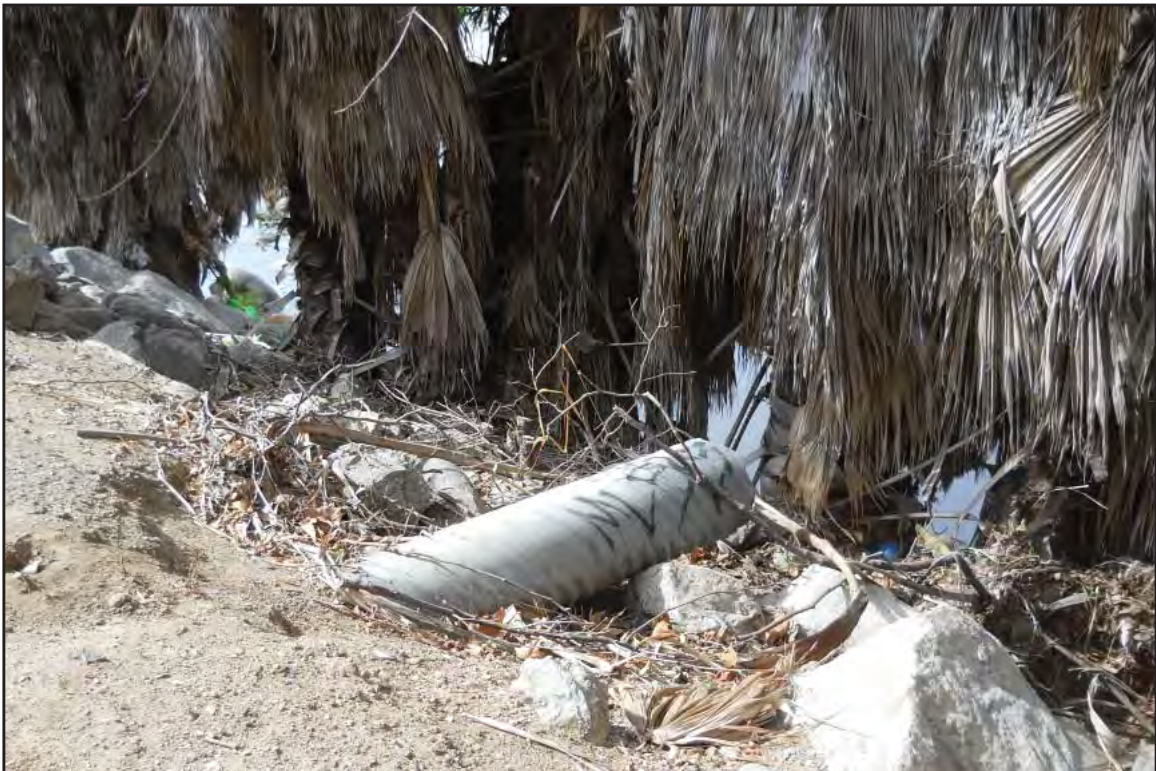
Photo B of Feature 13 Culvert, east of Laguna Channel, facing southwest
