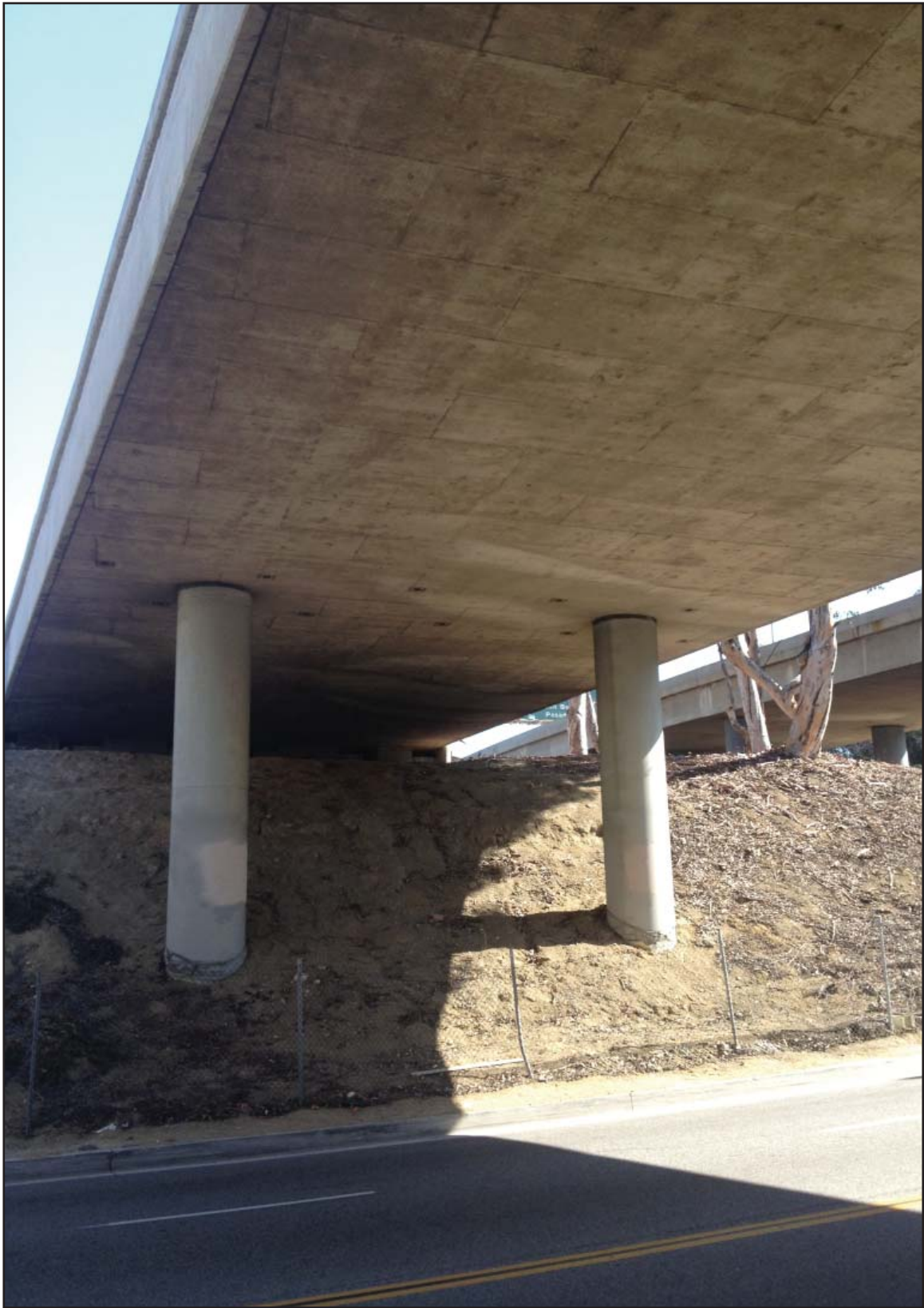
PHOTO 3 Ramona Blvd UC Bridge (L), facing north
