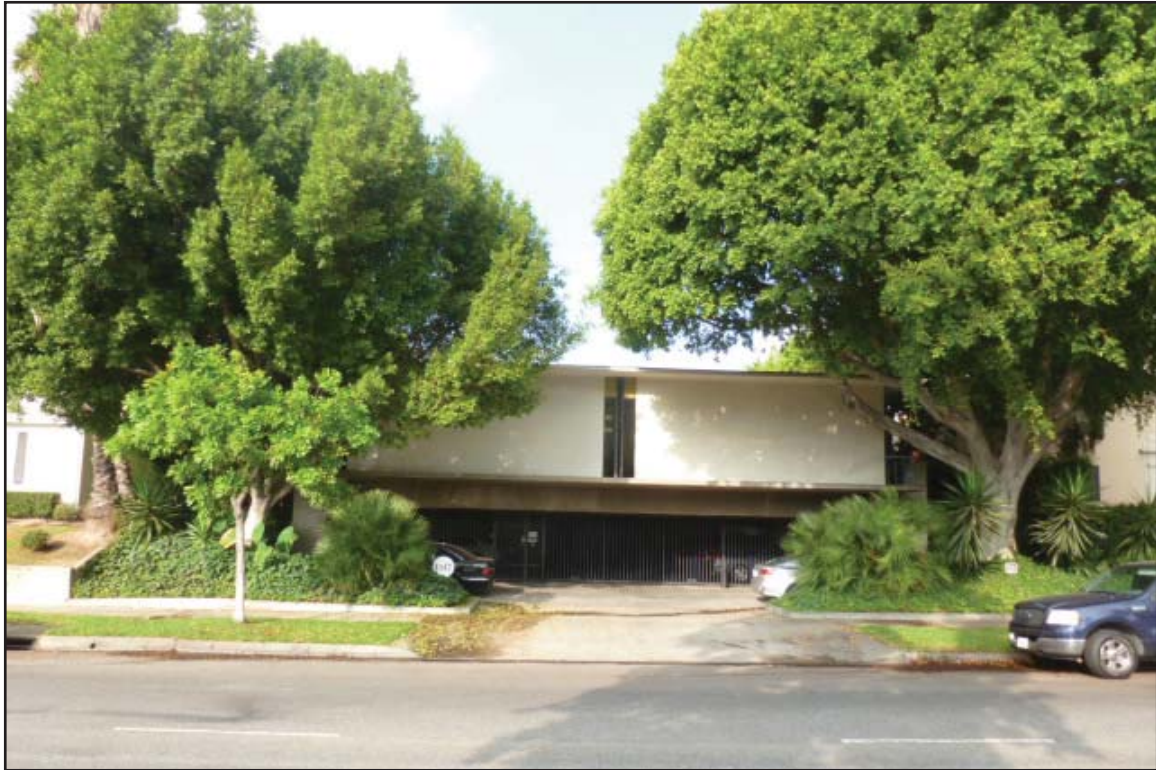
POINT COUNT LOCATION # 7 Looking West: (August 1, 2013)
