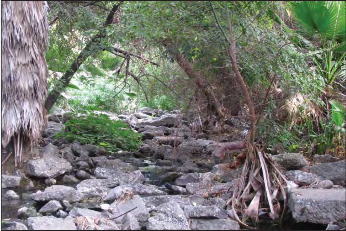
Photo A of Feature 15 Laguna Channel, underneath SR 710 and I 10 freeway interchange
