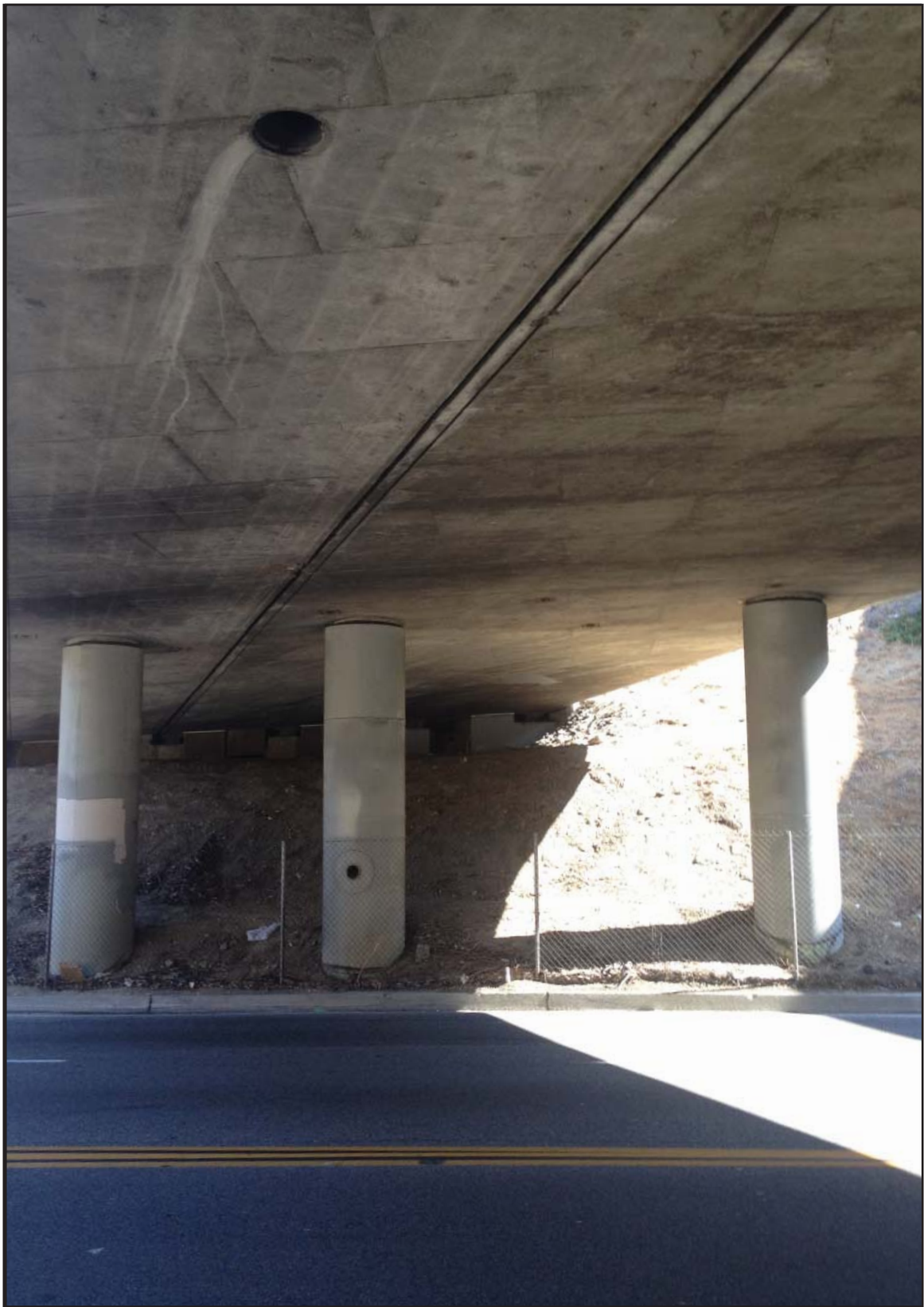
PHOTO 5 Ramona West Bridge, Facing North
