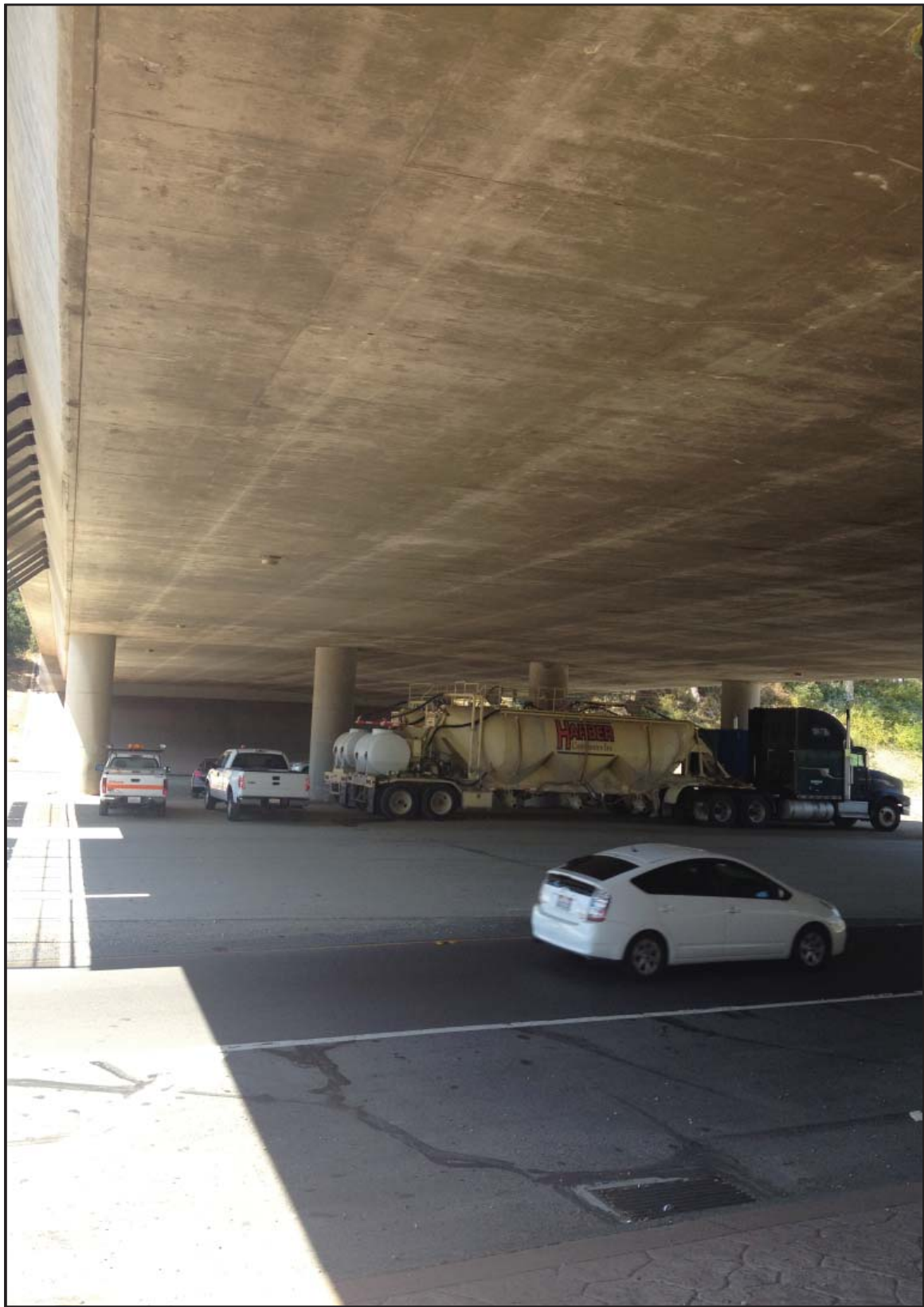
PHOTO 13 Del Mar Blvd OC Bridge, facing west: (August 29, 2013)
