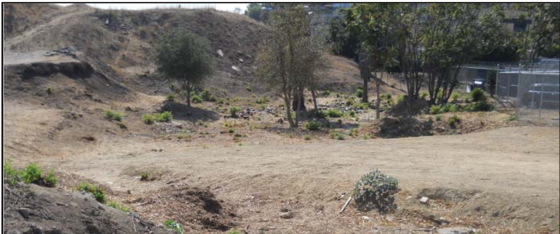
AREA 3 Looking West: (July 31, 2013)
