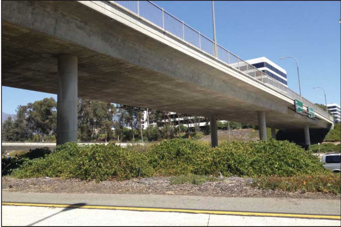
PHOTO 17 Union Street OC Bridge, facing northeast: (August 28, 2013)
