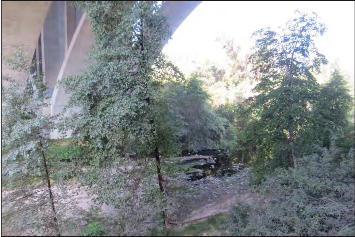
Photo C of Feature 5 Arroyo Seco under SR 134 bridge, facing north
