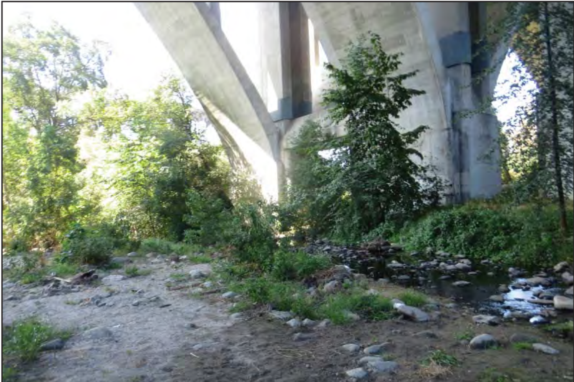
Photo D of Feature 5 Arroyo Seco under SR 134 bridge, facing south
