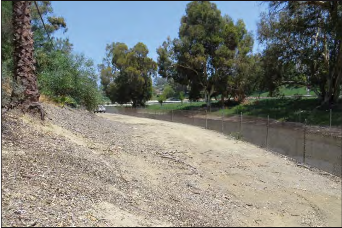
Photo A of Feature 11 Laguna Channel, west of SR 710, north of I 10, facing north
