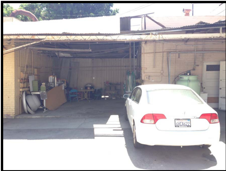
Photo 6: Middle of 1310 Fair Oaks building. Taken facing south.
