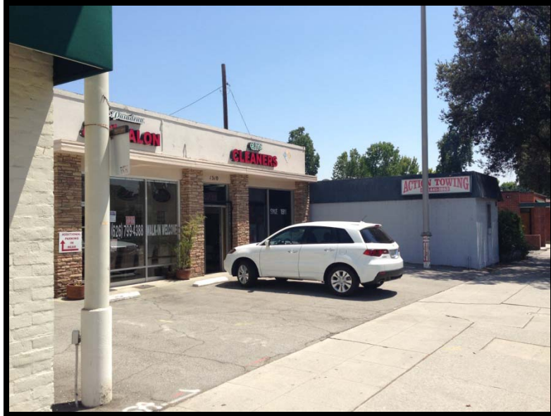
Photo 1: Front of Elite Cleaners. Taken facing southeast.
