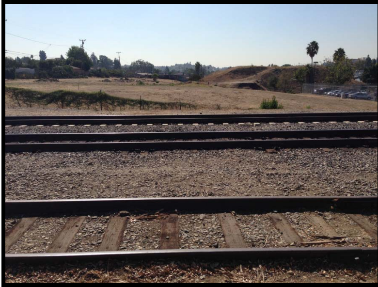
Photo 3: Railroad ROW. Taken facing south.
