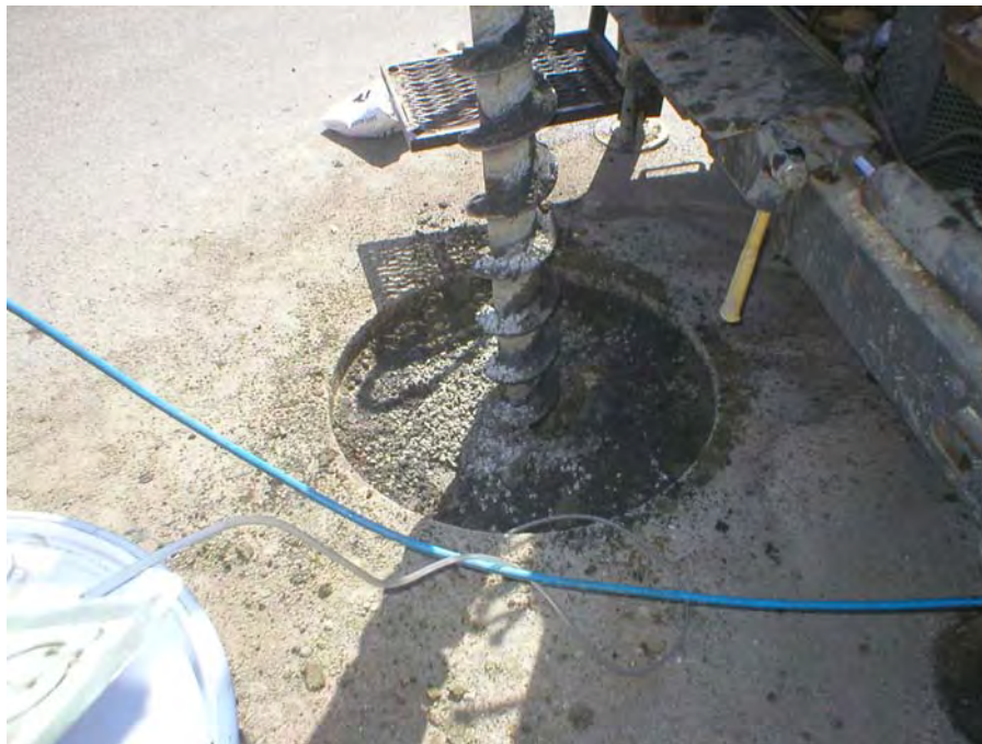
Photograph 12: Refuse encountered in LFG #5. Probe location was backfilled and sealed with bentonite chips.
