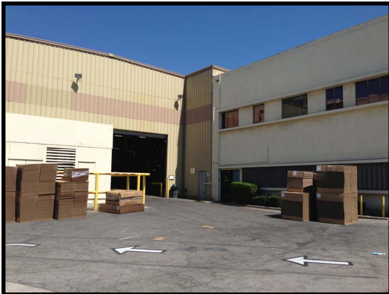
Photo 4: Loading docks. Taken facing northeast.
