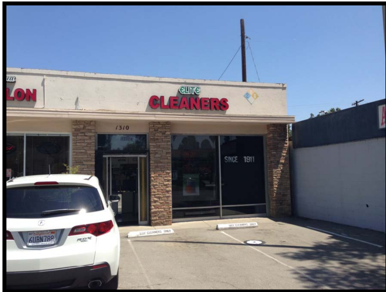
Photo 2: Front of Elite Cleaners. Taken facing east.
