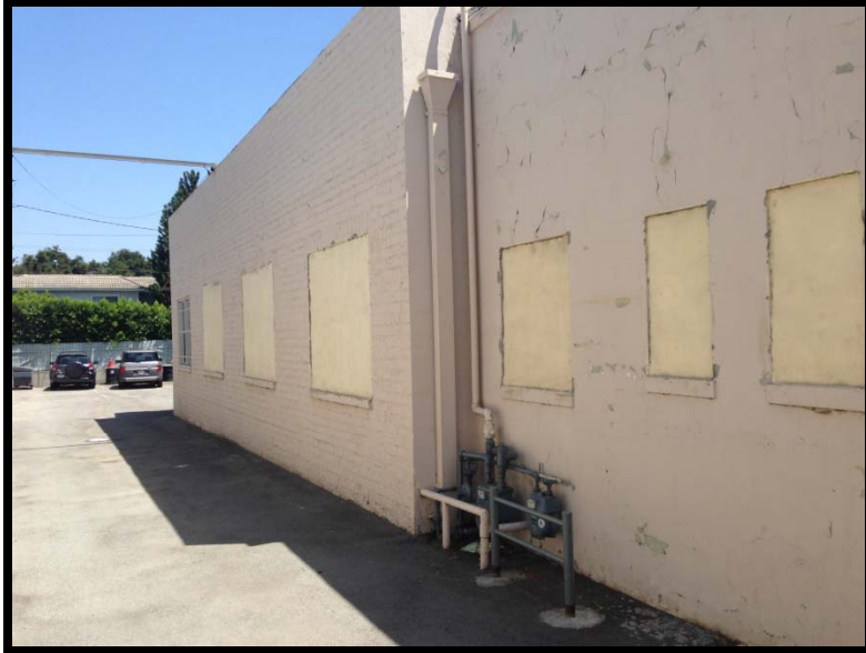
Photo 3: North side of 1310 Fair Oaks building. Taken facing southeast.
