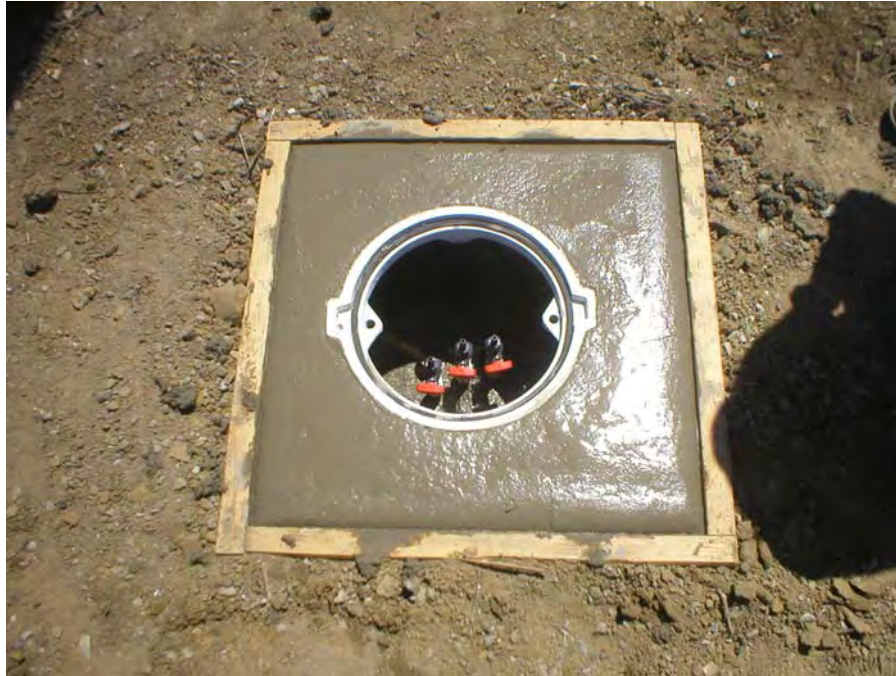
Photograph 13: Typical probe completion showing labcocks. In view is completed probe LFG #7.
