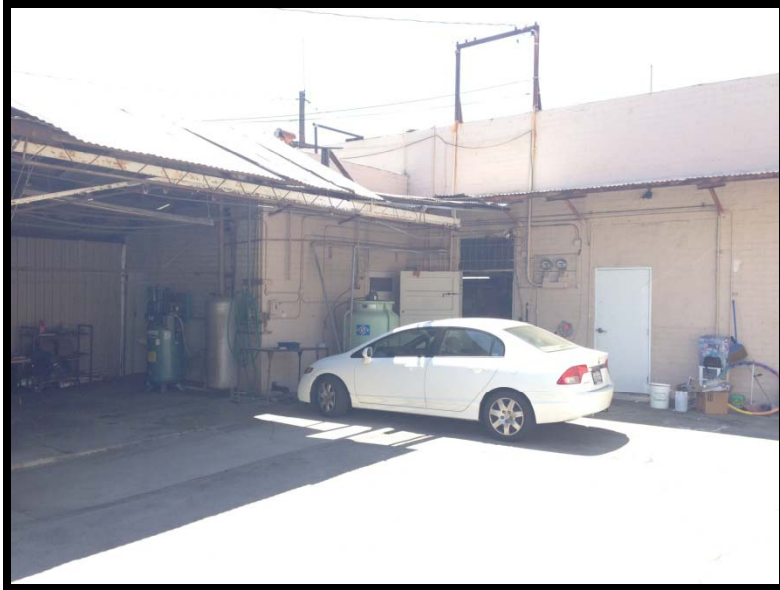
Photo 5: Middle of 1310 Fair Oaks building. Taken facing southwest.
