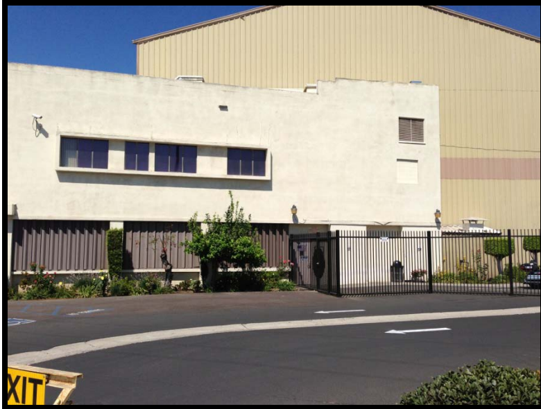
Photo 3. Office building. Taken facing north.
