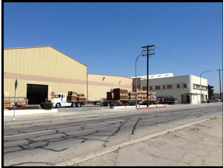
Photo 7. Mission Corrugated facility. Taken from across Mission Road facing northeast.
