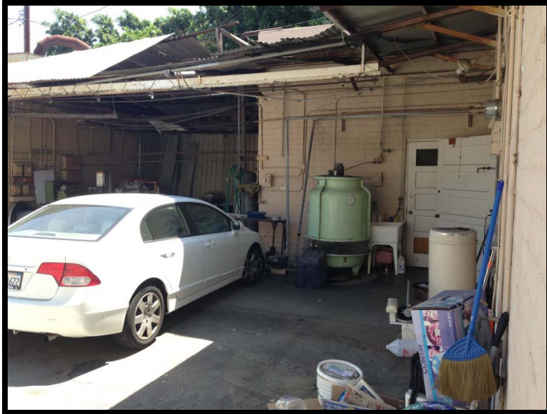
Photo 7: Middle of 1310 Fair Oaks building. Taken facing southeast.
