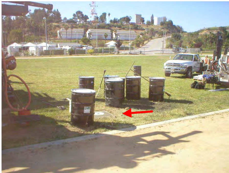
Photograph 10: Completed wellhead for probe LFG #4.
