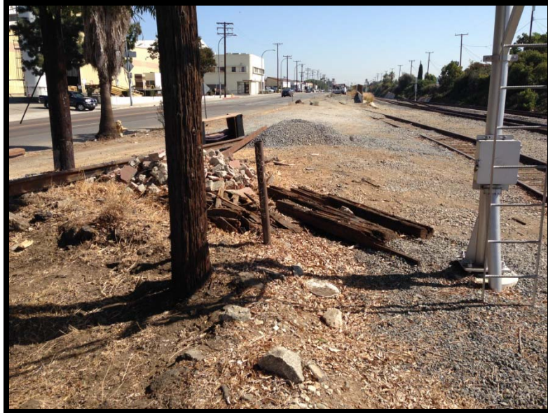
Photo 5: Pile of waste concrete and wood. No soil staining was observed near the piles. Taken facing east.
