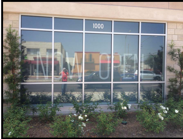
Photo 3: North side of bank. Taken facing south.
