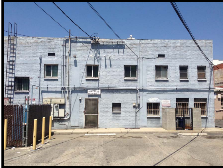
Photo 1: Rear of Fashion Master Cleaners. Taken facing north.
