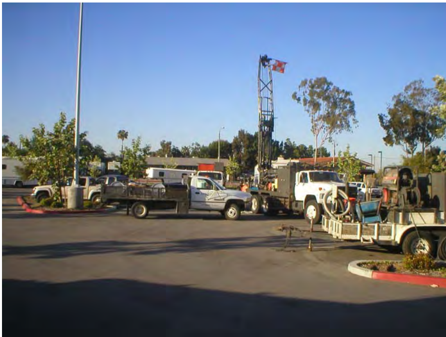
Photograph 2: Drilling LFG #1 using a hollow-stem truck-mounted drilling rig. This is a north facing view of the drilling operations associated with probe LFG #1.
