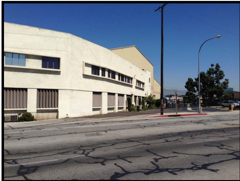
Photo 8: Office building. Taken from across Mission Road facing northeast.
