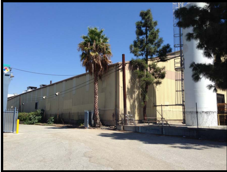
Photo 5. West side of Mission Corrugated facility. Taken facing northeast.
