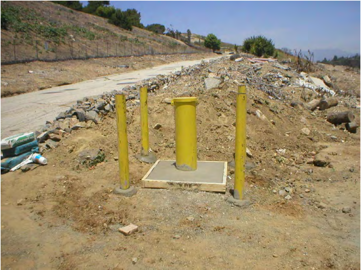
Photograph 16: Completed wellhead for well MW-1.
