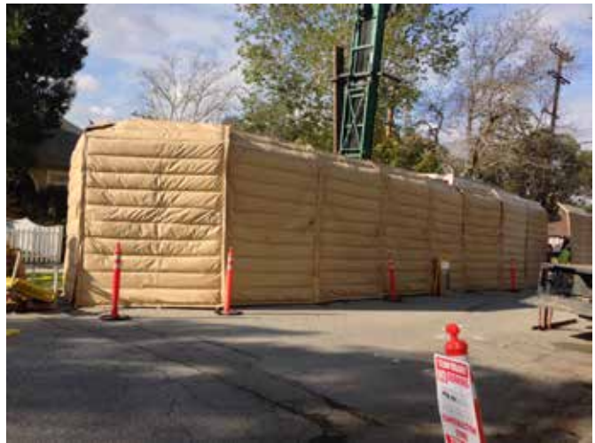
Figure 4. The sonic drill rig with the noise cancellation barriers in place.
