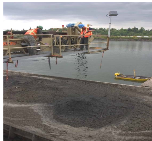
Consistency after being separated from slurry
