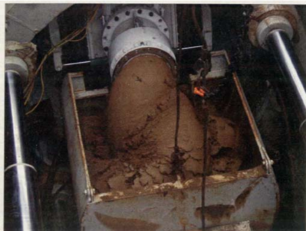
Excavated material being discharged from EPB TBM
