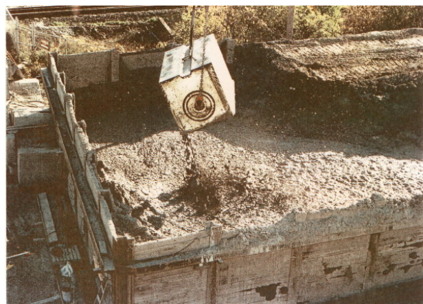
Excavated material consistency at surface after rehandling
