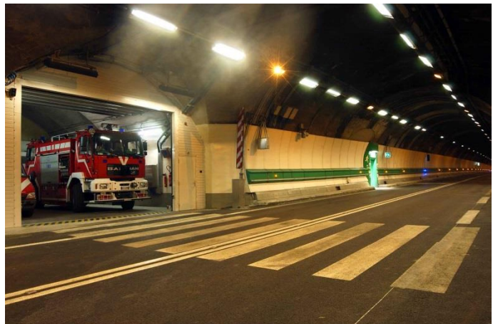
Figure 1 Mont Blanc Tunnel Fire Post
