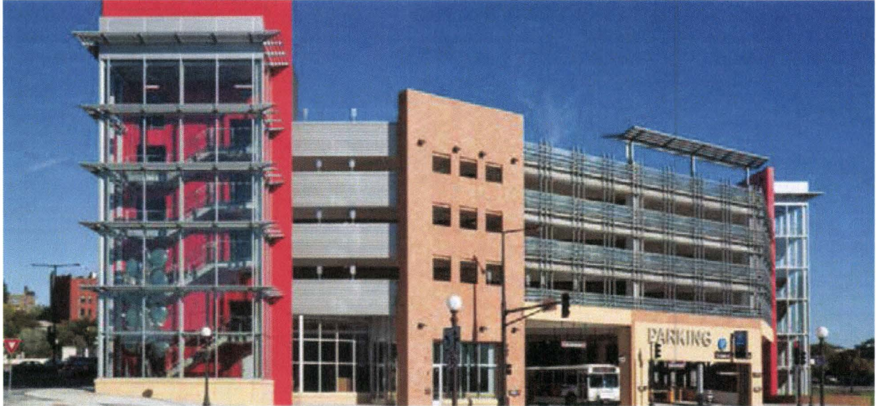
Exhibit 7. Example of Multimodal Transit/Parking Facility, Smith Avenue Transit Center in Saint Paul, Minnesota
