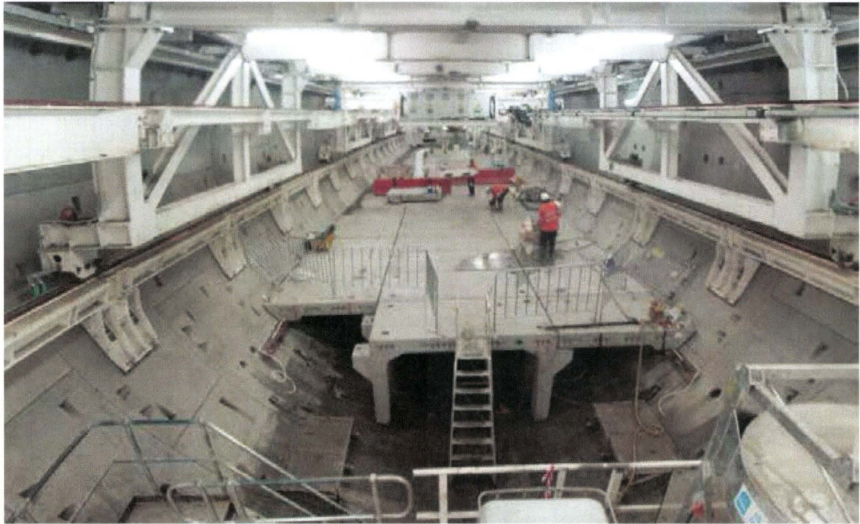
Exhibit 7. Brisbane Airport Link Tunnel Showing Installation of Single-Deck Precast Segments
