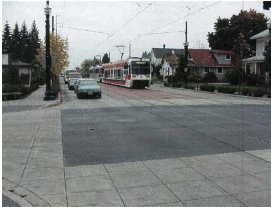
This photograph shows the TriMet LRT in the median of Main Street through the residential area of Hillsboro, Oregon. Although it may not exactly represent the potential LRT on Sheffield Avenue, it offers similar street geometry and traffic functions.
