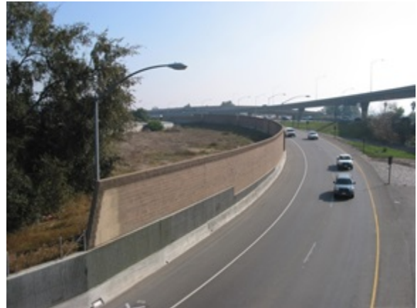
Typical Noise Barrier Along a Freeway
