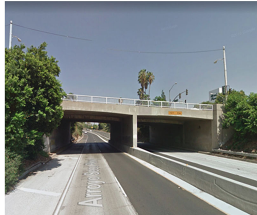
Figure 3.2-3: View of Fair Oaks Overcrossing Looking East
