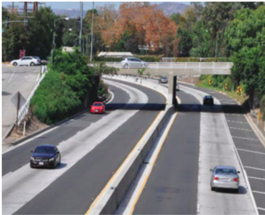
Figure 3.2-2: View of Dual-Tone Pavement, Looking East
