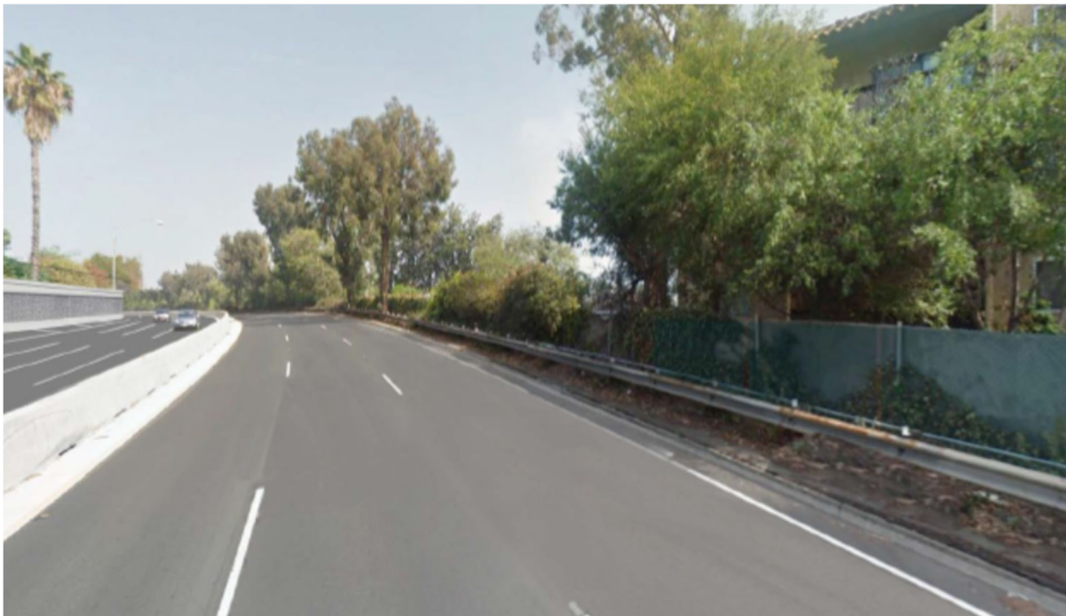
Figure 4.2-8: Simulated View Showing the Proposed TSM/TDM Improvements from SR 110 South of the Northbound Fair Oaks Exit, Facing North
