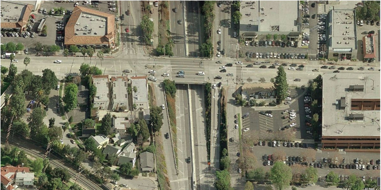
Figure 4.2-1: Existing Condition: Aerial Photo of the Fair Oaks Off-Ramp Exit from the Arroyo Seco Parkway, Looking East
