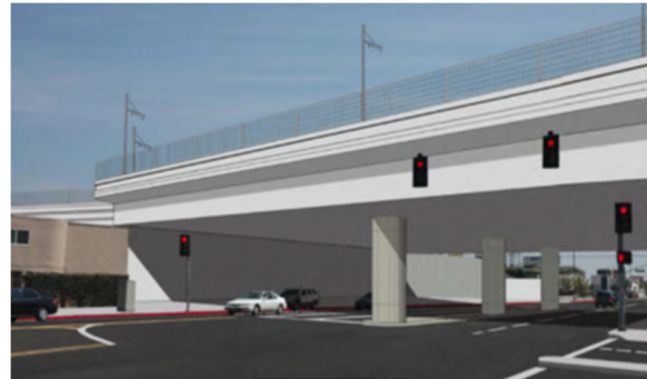
LRT Maintenance Structure at Valley Blvd
