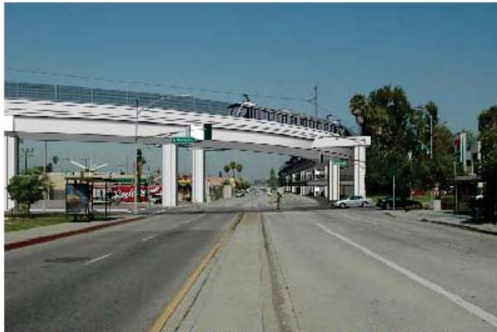
Visual Simulation: Light Rail Transit running above N. Mednik Avenue looking towards Floral Station.
