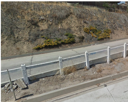
Figure 3.2-4: Contributing Curb and Gutter
