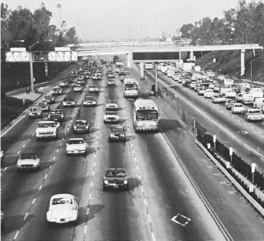
Buses and carpools in the exclusive high-occupancy "Diamond Lane" glide past slower traffic in the three regular lanes on the Santa Monica Freeway. The joint-agency project is scheduled to be evaluated over a one-year trial period.
