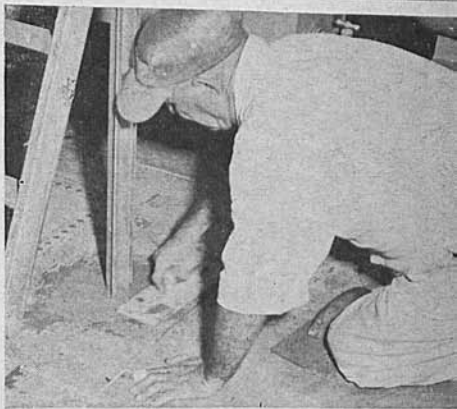
ABOVE — Saldivar loosens cement, while Leonard holds broom to stop flying pieces. UPPER RIGHT — New sign with new-type supporting pole is taken from supply on truck, placed in old hole, and ( RIGHT ) cemented in. Proper informational slats are then installed. INFORMATION SLATS are made in MTA shops. Here Harlan Schumacher is painting lettering on a sign at the South Park Shops.
