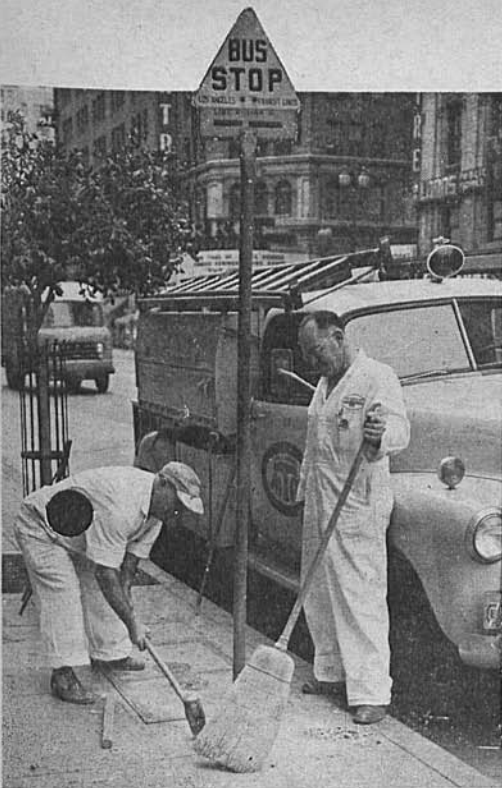
ABOVE — Saldivar loosens cement, while Leonard holds broom to stop flying pieces. UPPER RIGHT — New sign with new-type supporting pole is taken from supply on truck, placed in old hole, and ( RIGHT ) cemented in. Proper informational slats are then installed. INFORMATION SLATS are made in MTA shops. Here Harlan Schumacher is painting lettering on a sign at the South Park Shops.
