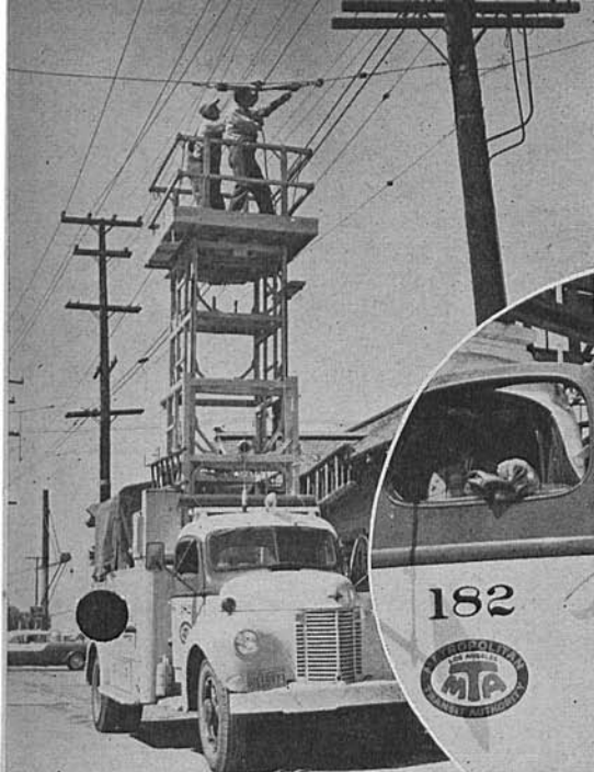
SOUTHERN DIVISION TOWER TRUCK — Tightening trolley wire and repairing broken span at Watts Substation. On tower are A. L. Rust, Leader, at left, and Manuel Montes, Lineman. Circled are Southern Division Line Foreman T. R. ("Dave") Foyle, right, and Driver-Groundman Norse Click, getting instructions from Mr. Foyle.
