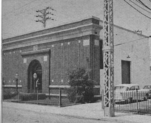
TYPICAL SUBSTATION — Slauson "Sub" (above), at Slauson and Towne Aves., with (picture at right) network of transmission lines and switches carrying voltages from 16,500 (as we buy it from the Edison Co.) down to 600 (what we use on trolley wires). Network is behind the substation.
