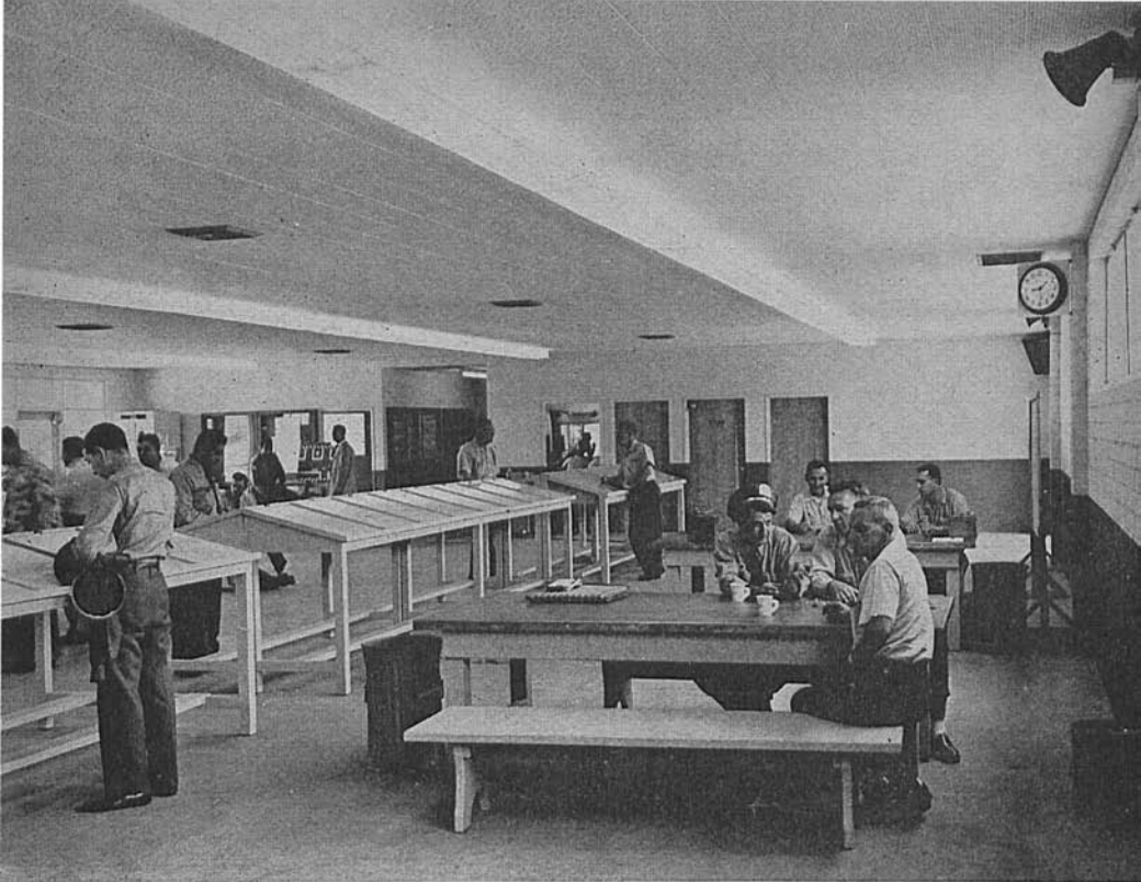
OPERATORS' WAITING ROOM —a view looking lengthwise, showing new furniture, new assignment tables, excellent and plentiful fluorescent lighting, acoustical tile in ceiling, public address system, etc. Opening in far wall at left center leads to washroom and locker room. One of the two main entrances is visible at the far left.
