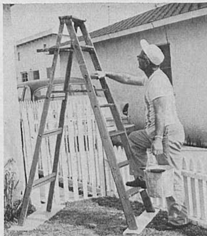
H. V. PRATT , Division 20 Operator, puts boards under ladder on soft ground before he climbs up to paint the eaves.
