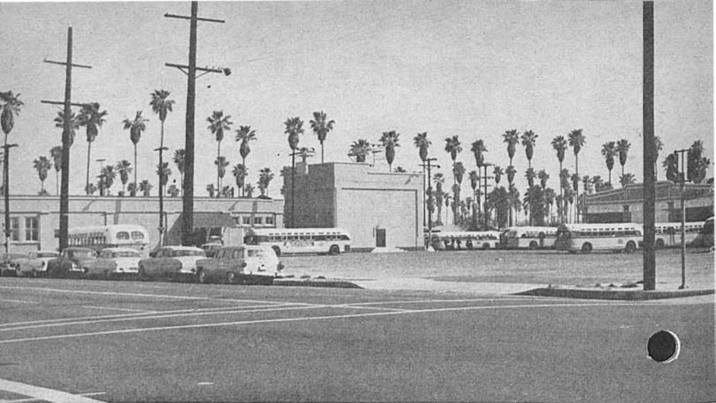
DIVISION 5, at 2300 W. 54th St., Los Angeles, as seen when one looks southeast from the corner of 54th St. and Second Ave. The transportation building is at extreme left. The taller, square building is an electrical substation which supplies the current for
