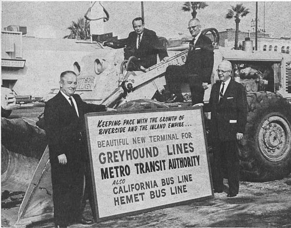
BULLDOZER REPLACES SHOVEL AT GROUND-BREAKING —Participating in Oct. 5 ceremony announcing the start of construction of new station in Riverside for Greyhound, MTA, Hemet Bus Line, and California Bus Line, are: in driver's seat, C. D. Kirkpatrick, Vice-President, Marketing, Western Greyhound Lines, San Francisco office; on bulldozer step, Thomas N. Bristow, Supervisor of Stations and Agencies, MTA. On ground, from left, are Lewis F. Crosby, Agent; and R. O. Christiansen, Director of Public Relations, MTA.
