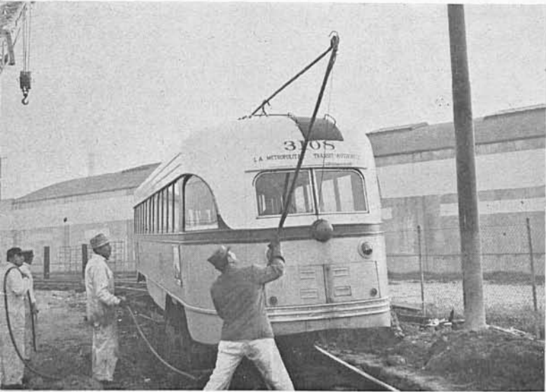
UPPER LEFT—Streetcar waits near entrance to Vernon Yard while Way and Structures crew under Foreman Harvey Lindley lays a lead track (UPPER LEFT, UPPER RIGHT) to connect with storage track. As soon as one storage track was full, the lead track was moved to connect with the next storage track. LOWER LEFT—Since there is no overhead trolley wire beyond a certain point on the lead track, a crew carries a 300-foot flexible 600-volt power cable
