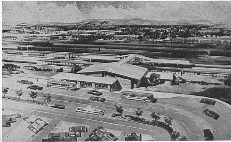
SURFACE STATION for rapid transit system, showing park-and-ride, kiss-and-ride, and feeder bus line facilities. An artist's sketch.
