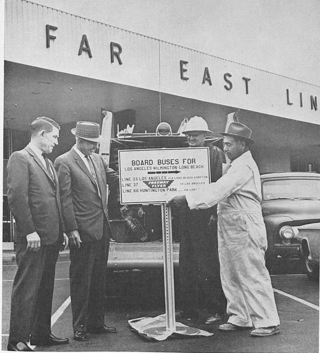
STOPS AND ZONES crew bolts to a portable standard a directional sign for boat passengers, as other interested MTA men look on. Left to right are W. C. Weimer, Community Relations Representative, who helped decide where the signs (there are two) should be placed; L. S. ("Cappy") Hendricks, Representative, Stops and Zones; and the crew, Carle Heffington and Jose Aguirre. The scene is the parking lot for the new passenger building on Pier 93, at the Los Angeles Harbor.
