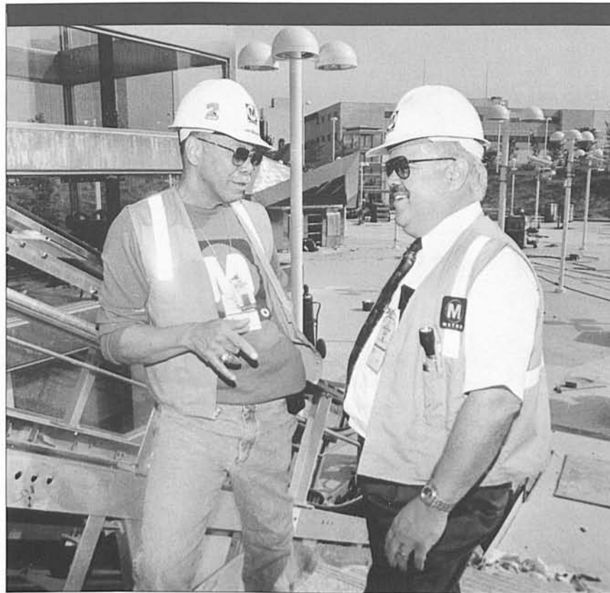
Jack McDowell (L) of MTA Construction and Jesse Diaz of MTA Rail Operations are working together to bring the Wilshire Line into service this July. The Wilshire/Vermont station plaza, nearing the end of construction, is shown in the background.
