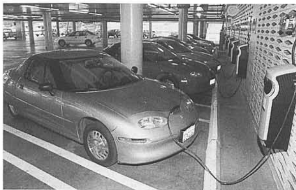
A General Motors EV1 electrical vehicle takes a power charge at a multi-bay charging station at DWP headquarters in downtown LA. A similar charging station will be installed soon at MTA Headquarters.
