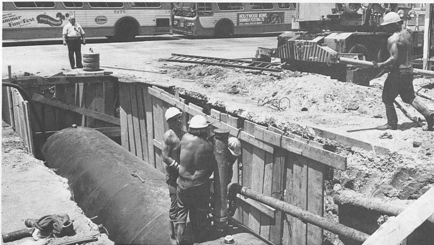
HANDLE WITH CARE —The crew of the building and grounds section recently installed a 10,000-gallon fuel pump at Division 7, replacing a ruptured one.
