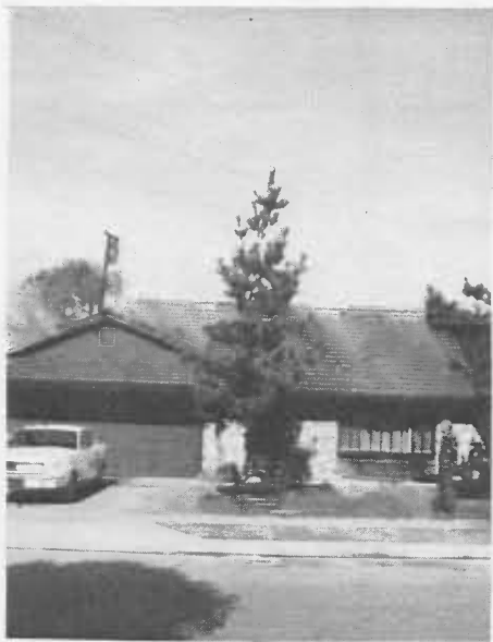
This is how Franklin's house looks after he remodelled it.
