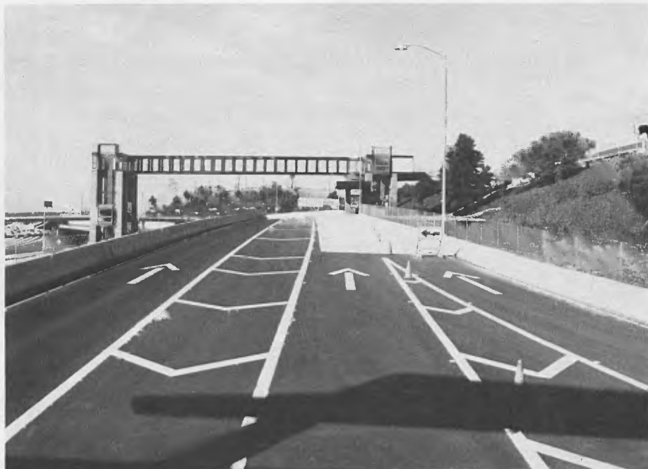
A view of the station from a westbound El Monte bus. The left lane is for through buses; the center lane is for arriving buses at the westbound platform; and the right lane is an on ramp from southbound Long Beach Freeway.
