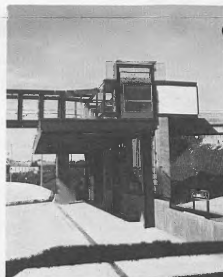
A close-up view of the westbound loading platform at the Cal State Station on the El Monte Busway. The platform is 60 feet above ground.
