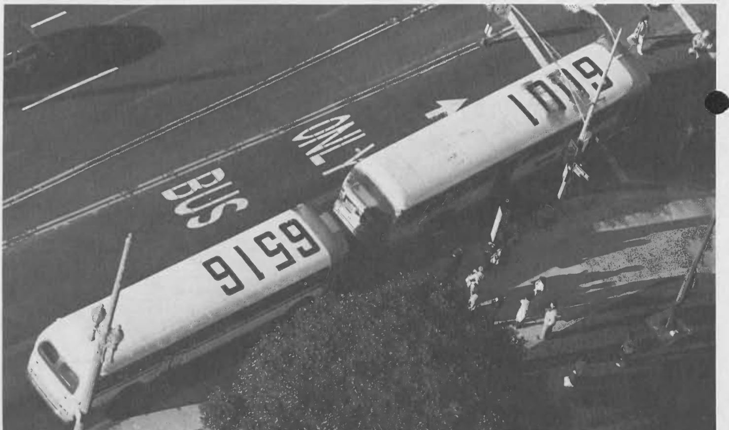
AFTER — Addition of extra lane, combined with splitting of busway and local stops, should alleviate crowding and give buses bypass capability in the event of breakdowns or traffic congestion.
