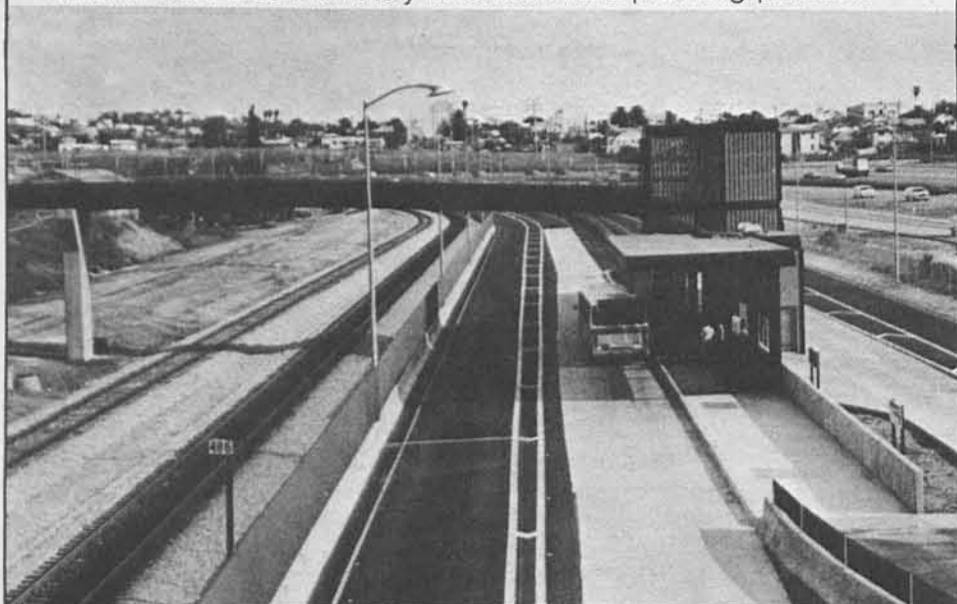
HOSPITAL STATION—Just one of three stations along the El Monte-Los Angeles Busway.
