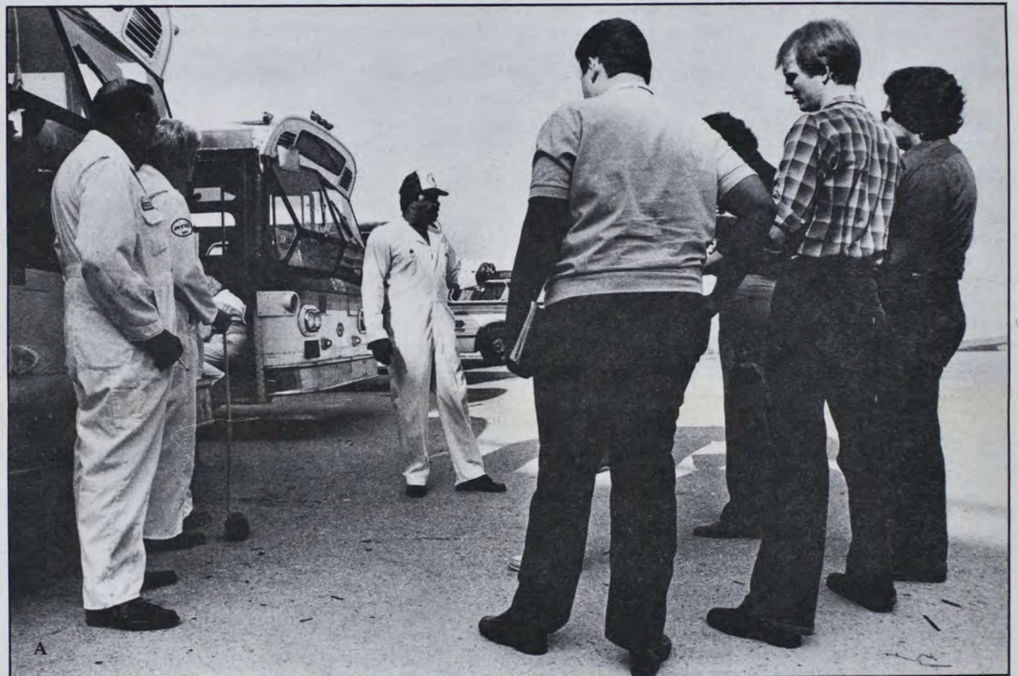
Photo A: Instructor Joe Singleton asks first-day trainees to estimate and write down the distance to bring a 30-mph bus to a full stop. Later, each trainee will perform the test and compare the estimate to the real distance required.
