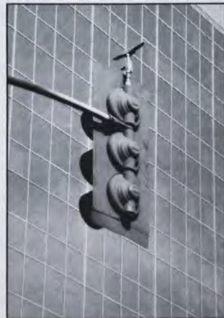
A state-of-the-art device developed by 3M Opticom System mounted on a traffic signal provides for green lights whenever a bus reaches an intersection along a 10-mile route of Ventura Boulevard.
