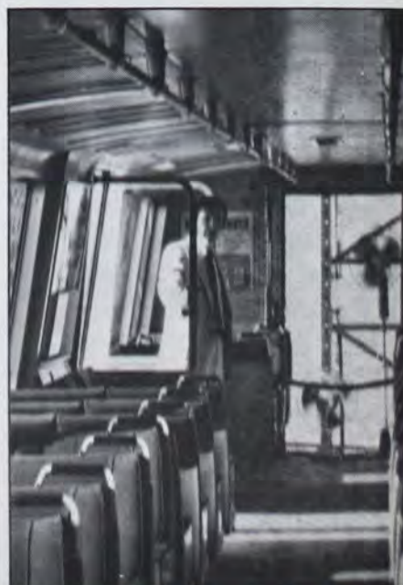
Mike Barnes explores the interior of the rail car borrowed from BART for the groundbreaking ceremony.
