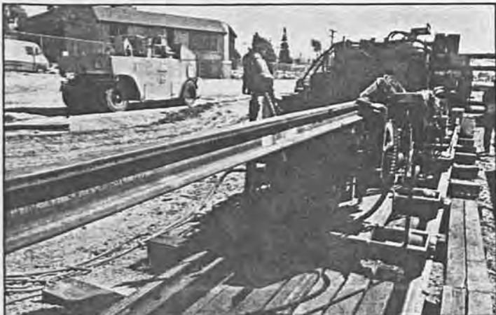
A 78-foot length of rail is readied for the welding operation.
