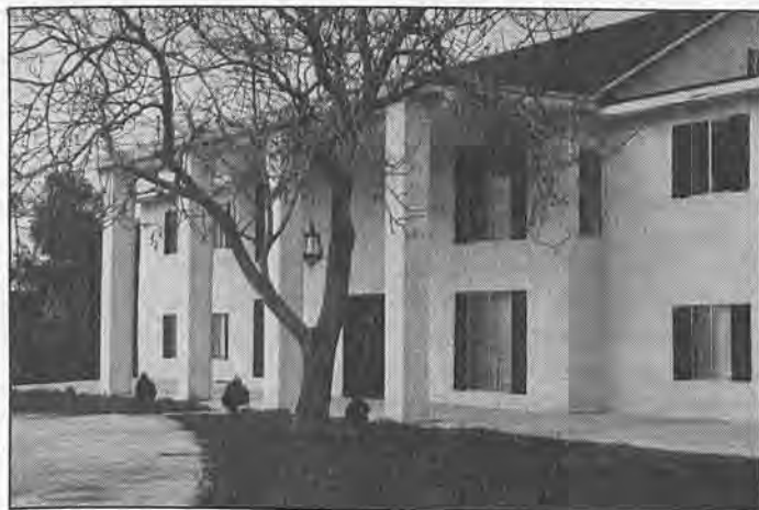
The front view of Operator George Pepper's Southern Colonial home in Fontana. Pepper built the house from scratch at an approximate cost of $64,000. His house was recently appraised at a value of $205,000.
