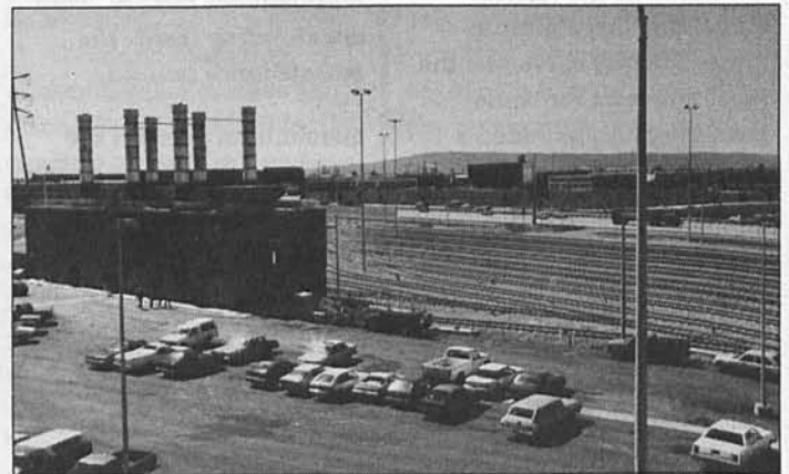
Looking like a Mississippi Delta Queen stands the Paint Shop rising above the rails in the yard.
