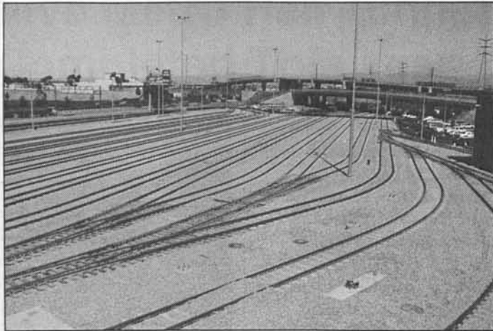
The light rail main yard is next to the Long Beach Freeway on 208th Street, one block east of Santa Fe Avenue. Here is an aerial view of the criss-crossing lines in the yard.
