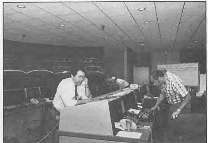
OCS Superintendent Dan Ibarra stays plugged into the system and is able to make his quick decisions based on the flow of information through the Supervisory Control and Data Acquisition (SCADA) system. TOS Gerald Harper (right) closely monitors his computer and makes operations adjustments after another message has been received in the command center.
