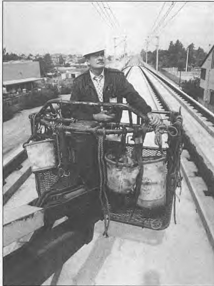
Rail Facilities Superintendent Walter "Bud" Moore checks the aerial cables that will propel the Blue Line trolleys along 22 miles of track between Los Angeles and Long Beach.
