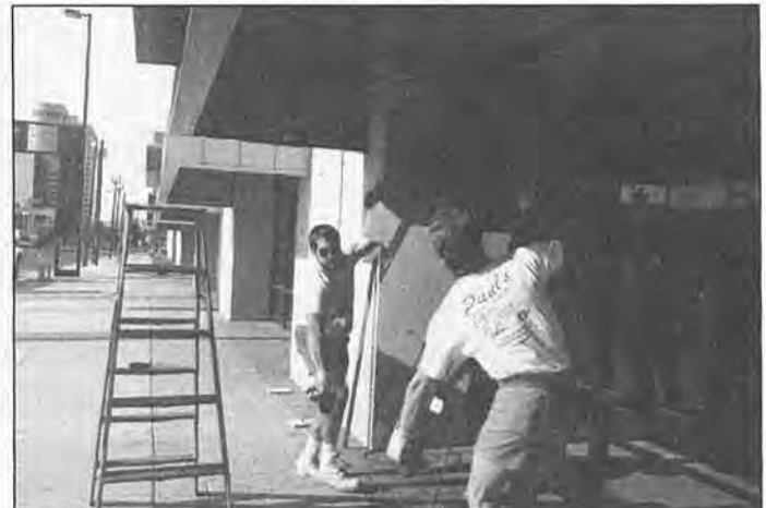
Workmen prepare the opening for the bus' entrance.
