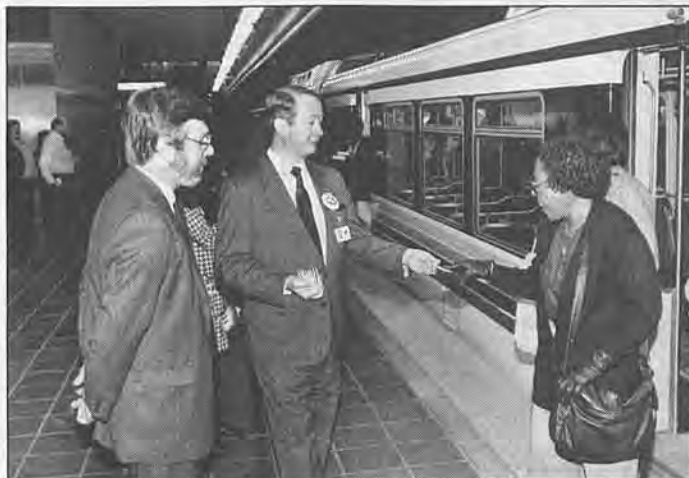
On opening day, General Manager Alan Pegg and Assistant General Manager Art Leahy greet patrons as they arrive at the station.
