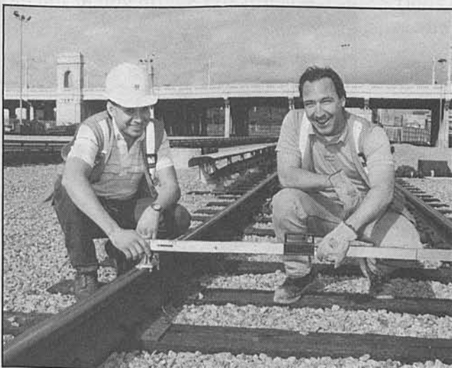
Track inspectors Ramon Alatorre and Mark Germanowski inspect the track for the proper gage.
