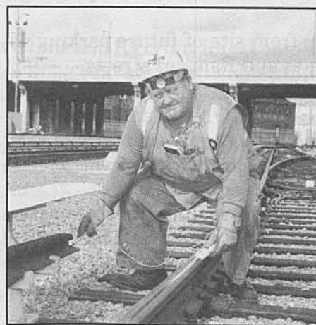
Traction power inspector Art Siemens tests for 750 volts of direct current on the rails.
