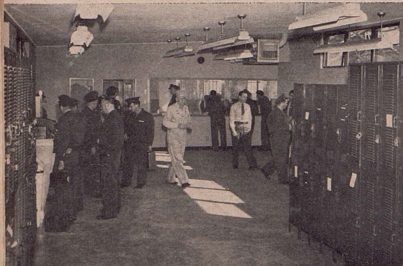
OPERATOR'S ROOM, looking from locker end toward the office of the division foreman. Pattern is similar to that at Van Nuys.
