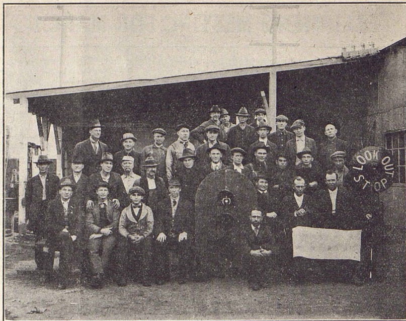
THE SIGNAL DEPARTMENT These Fellows Make Speed With Safety Possible
