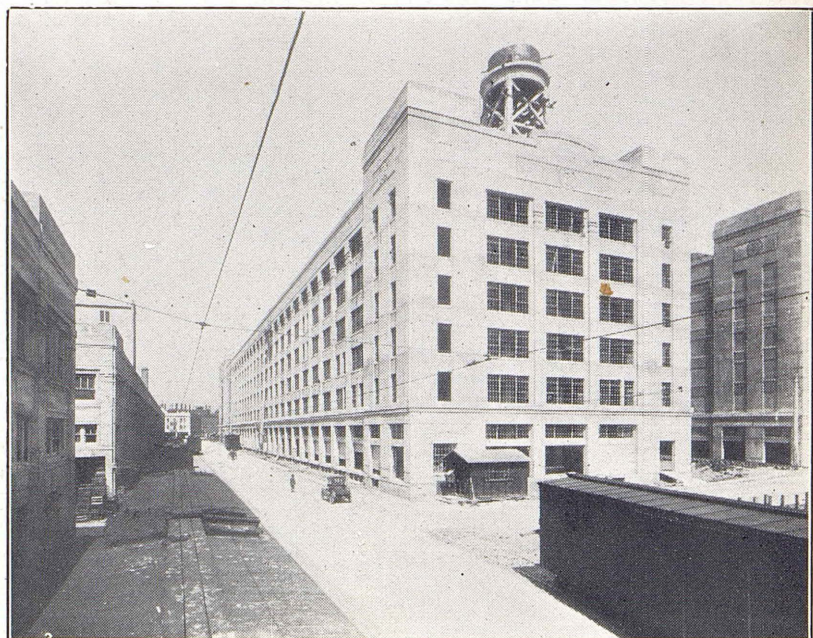
Sectional View of the Los Angeles Union Terminal Served Only by Pacific Electric Railway
