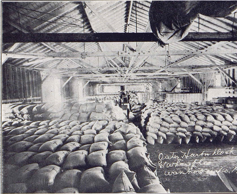
One Hundred Thousand Sacks of Cement, Moved by Pacific Electric, Being Stored in Outer Harbor Warehouse for Export
