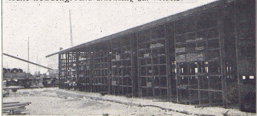
No.8—View shows a section of the Store Department's Iron Storage Rack, featuring the efficient storage of this class of material. Observe Store Department's Crane in background unloading Car Wheels.
