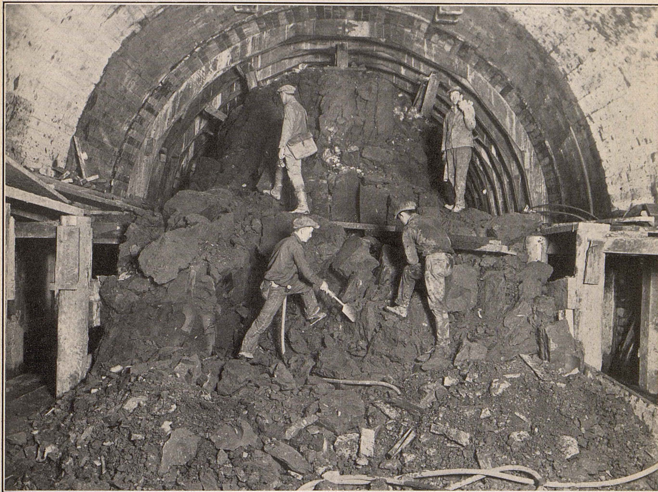
At one of the three faces of our great traffic bore. The work of excavating is advanced by sections, tunnel being divided into five sections, or drifts, and earth from each is removed in progressive order, the core being the last portion removed. At the time of taking this picture removal of supporting arch timbering and core was in progress.
