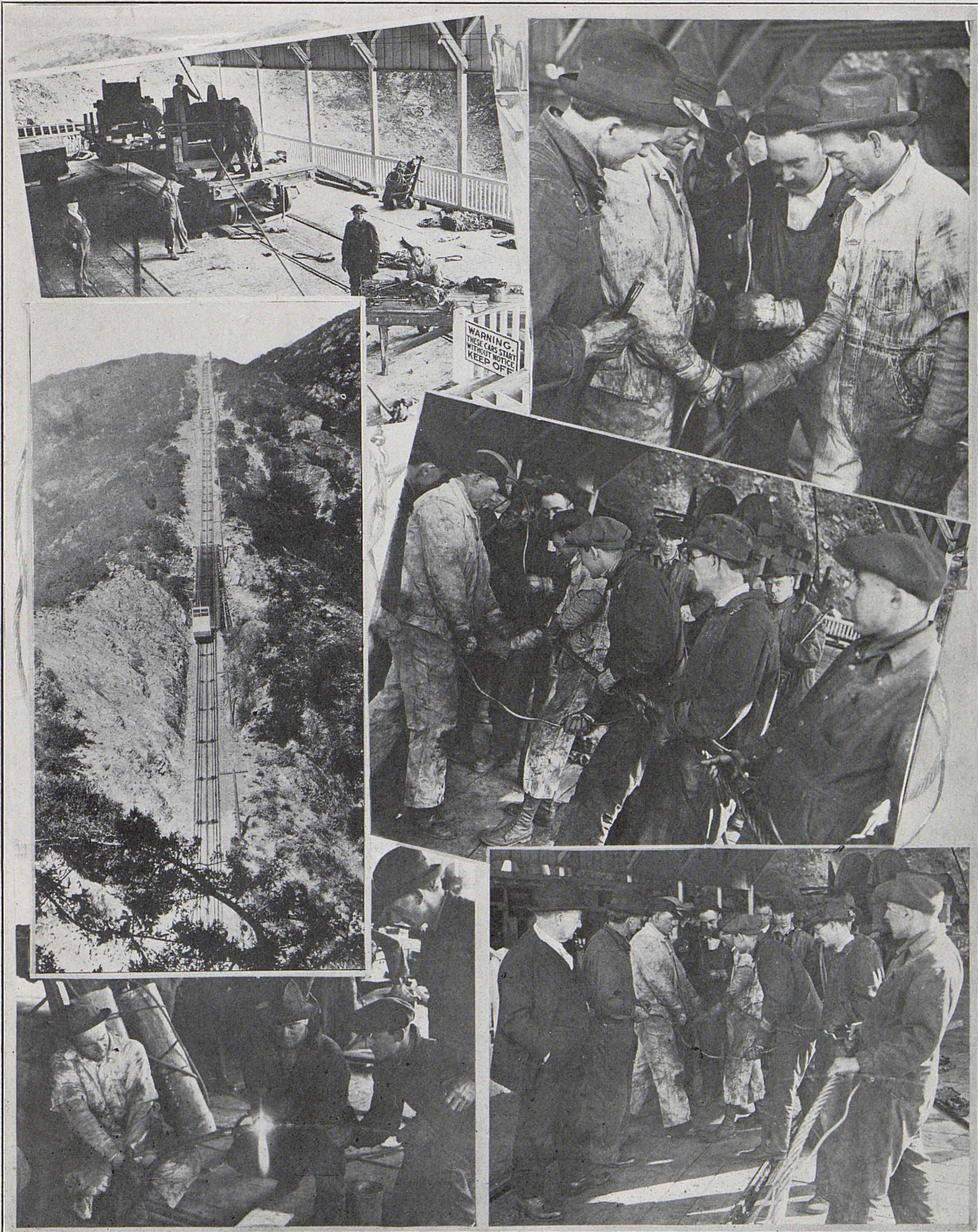
Snap-shot highlights during the replacement of Mt. Lowe pulling cable.
